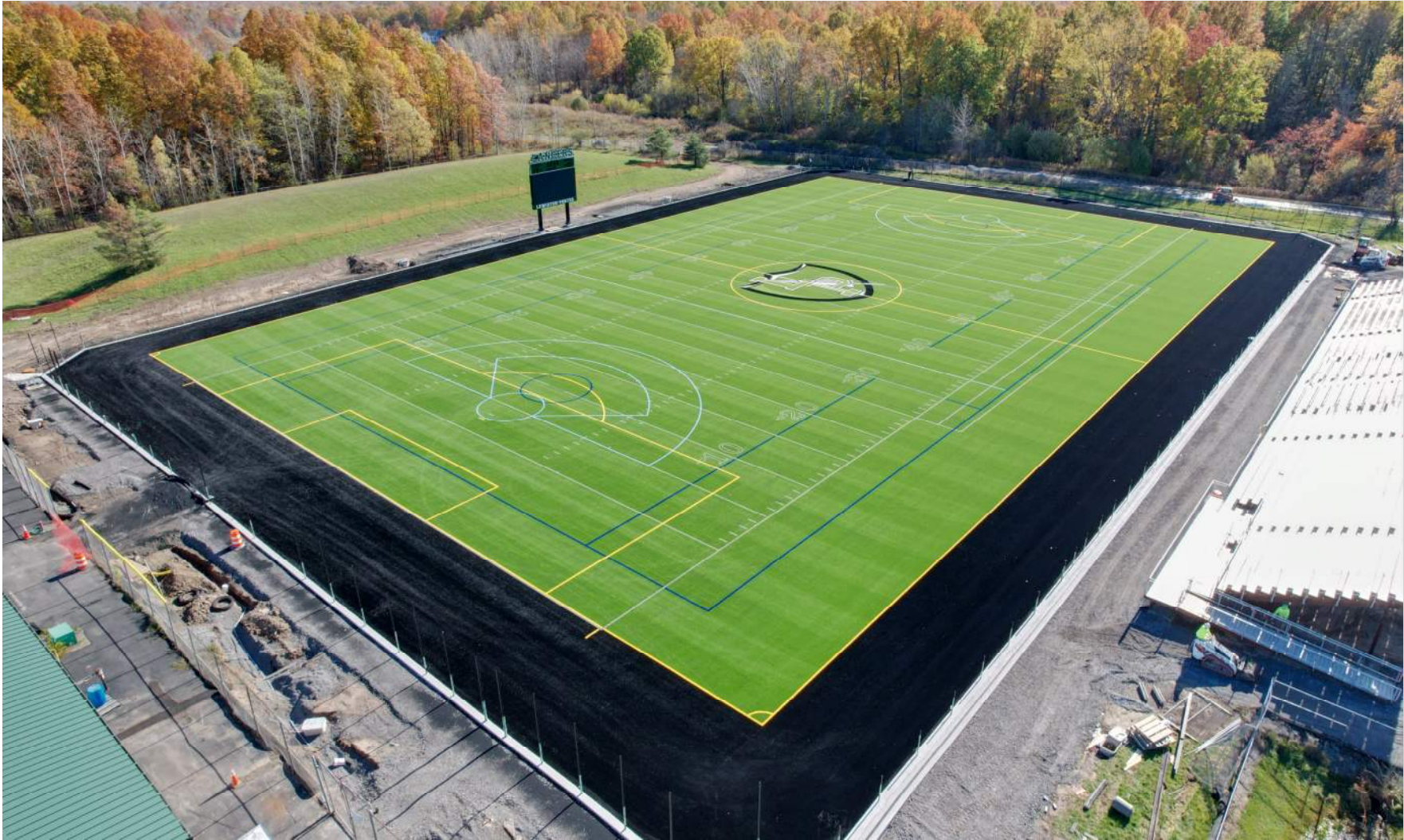
2024 CIP – Phase II Elia Stadium
