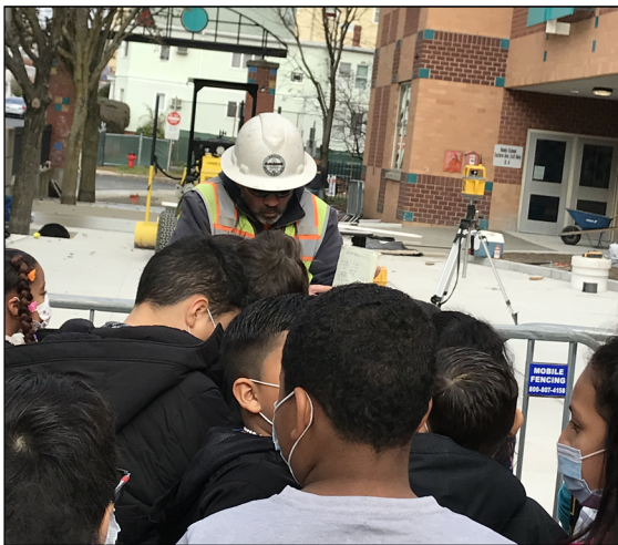
Third grade Sokolowski students visited the construction site outside the MCB Complex to learn about how area and perimeter are put to use. Students got to meet some of the workers, learn about survey equipment, review plans, and ask questions. Thanks to Chris from Argus Construction for coordinating with our school!
