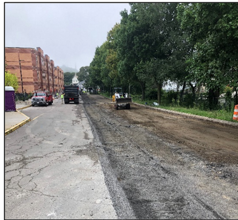
MCB Busway Paving
