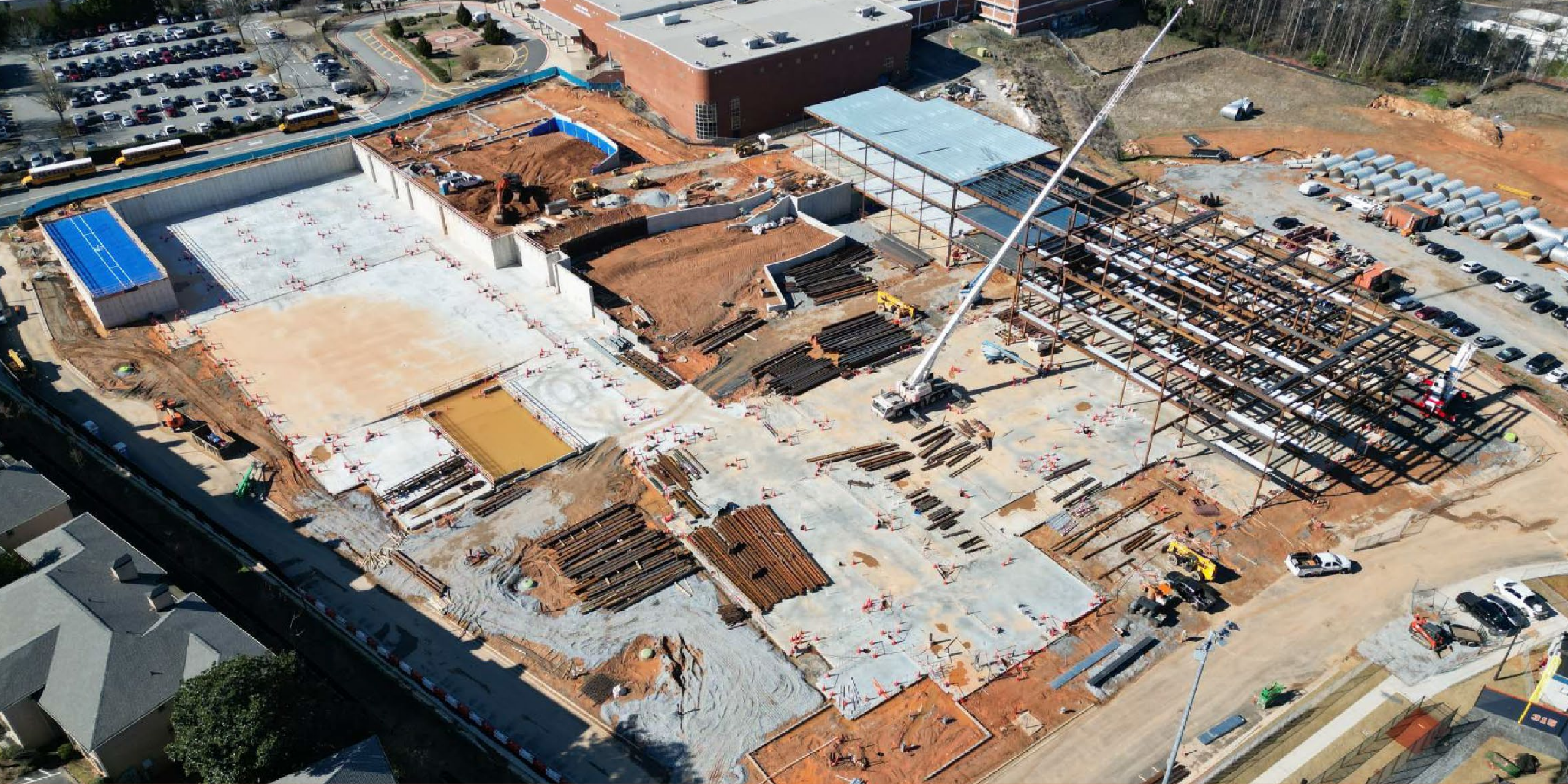
Overall aerial view
