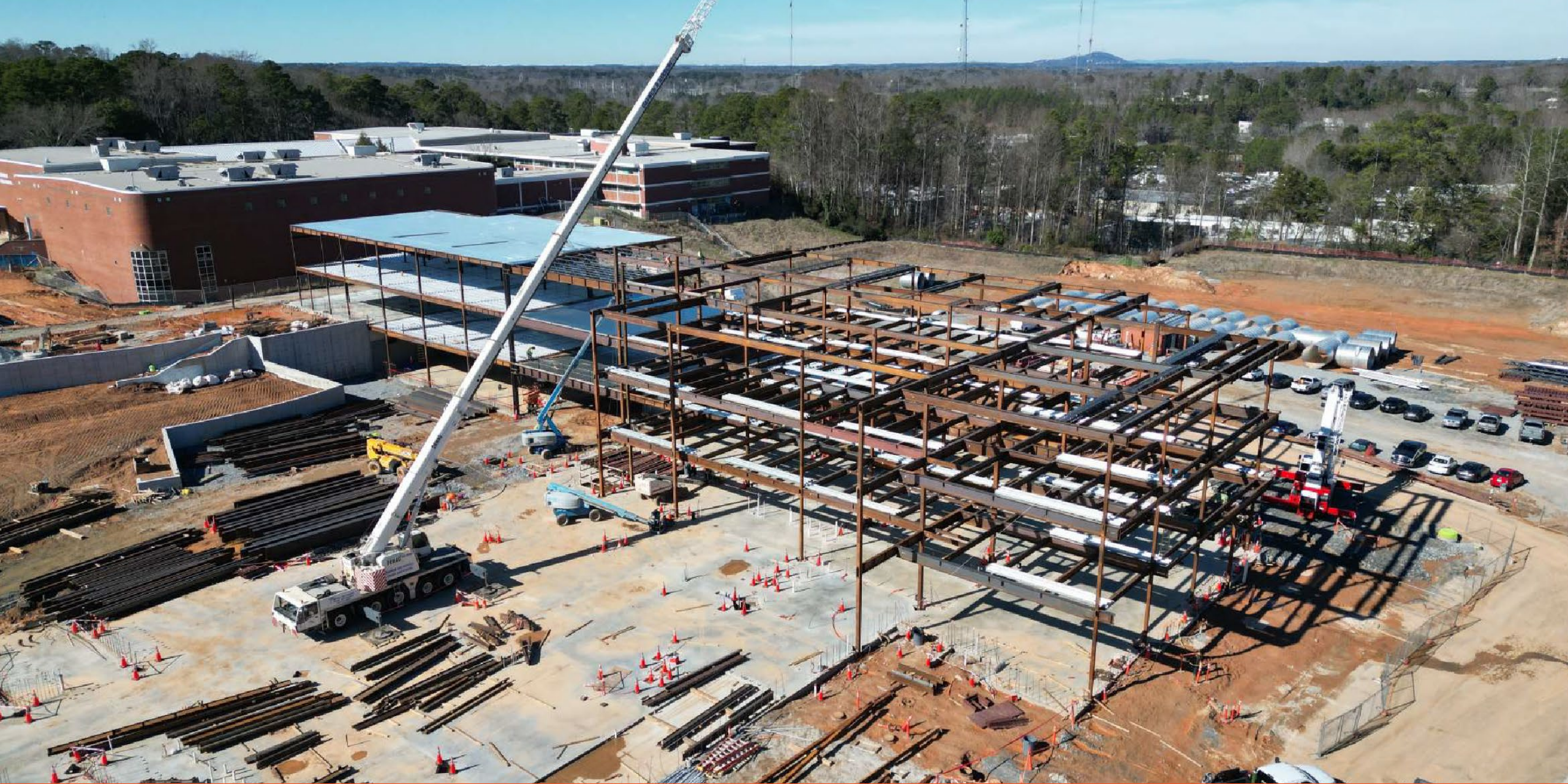
Main building progress
