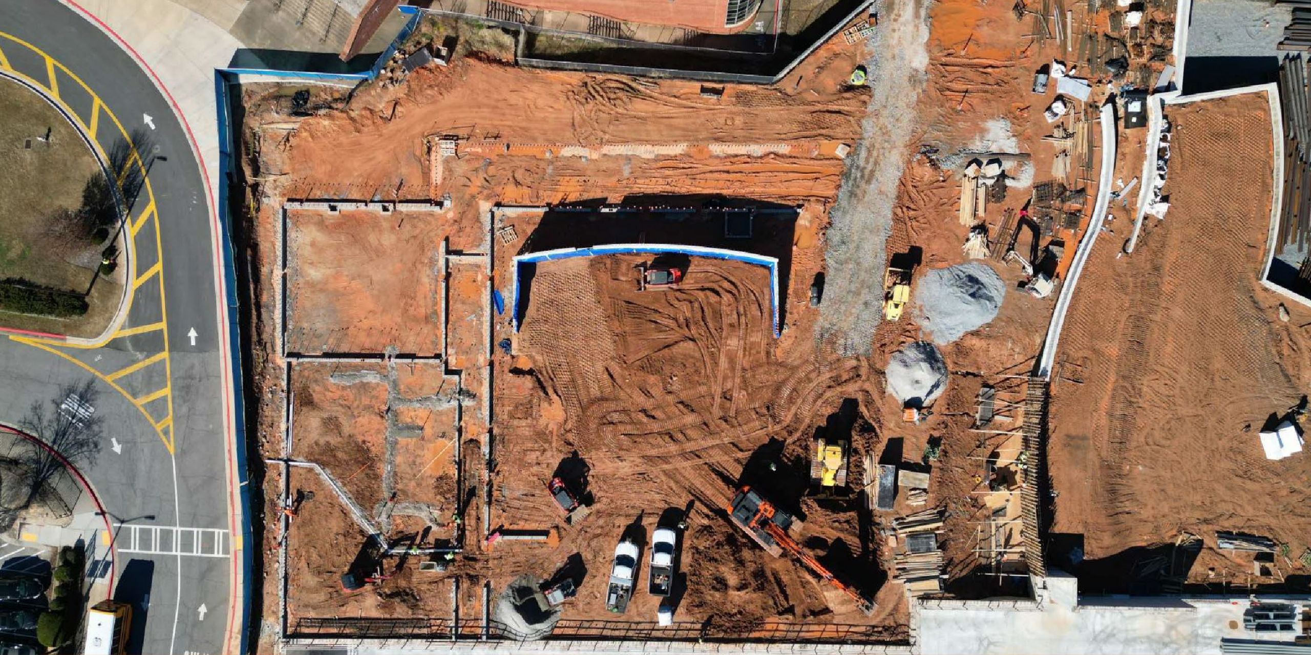
Performing arts foundation progress
