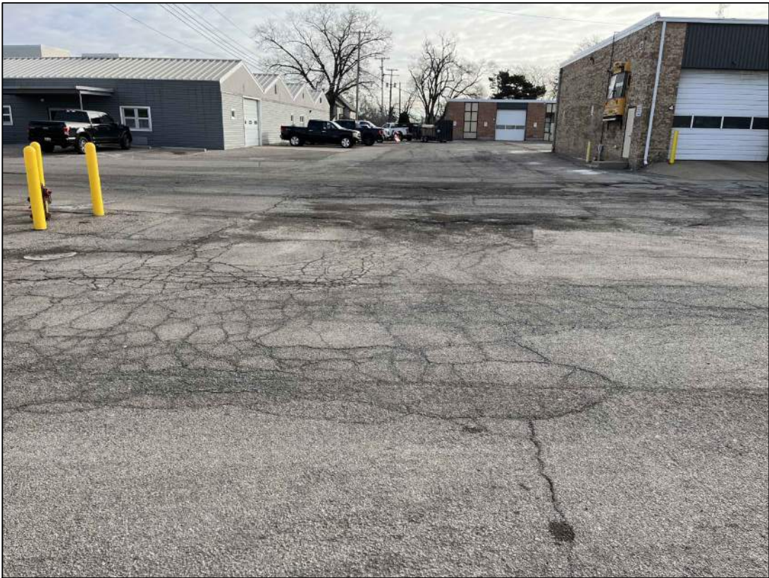
3 Block Cracking - Alligator Cracking - Potholes NTS
