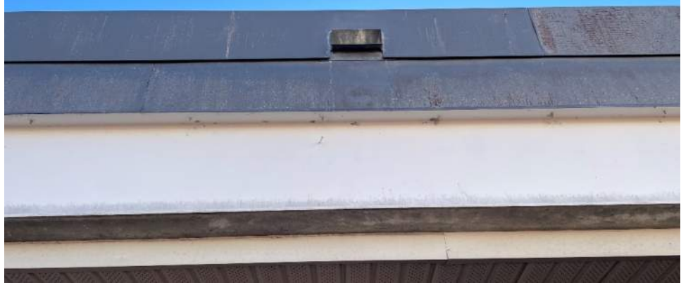
A field fashioned roof scupper in the metal fascia.
