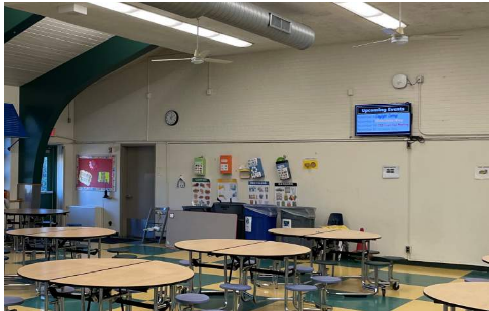
Wall mounted digital signage within the cafeteria.
