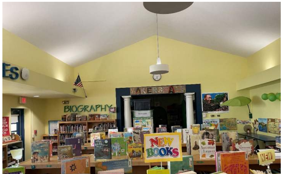
The vaulted gypsum board ceiling above the Media Center.
