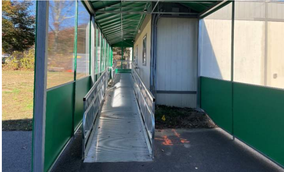
A view of the accessible ramp leading to the elevated entrance of the portable classrooms.
