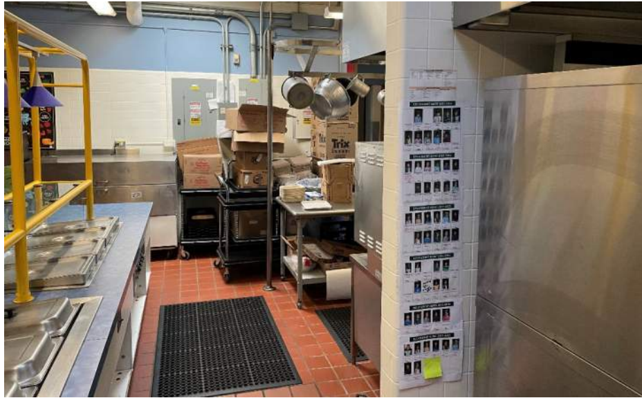
An example of the quarry tile floor finish within the Food Prep area.
