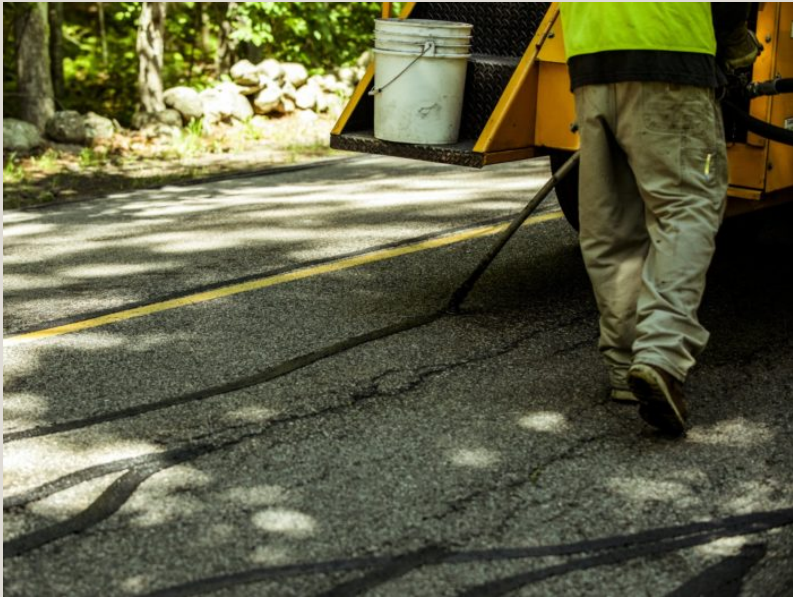
CRACK/MASTIC SEALING
