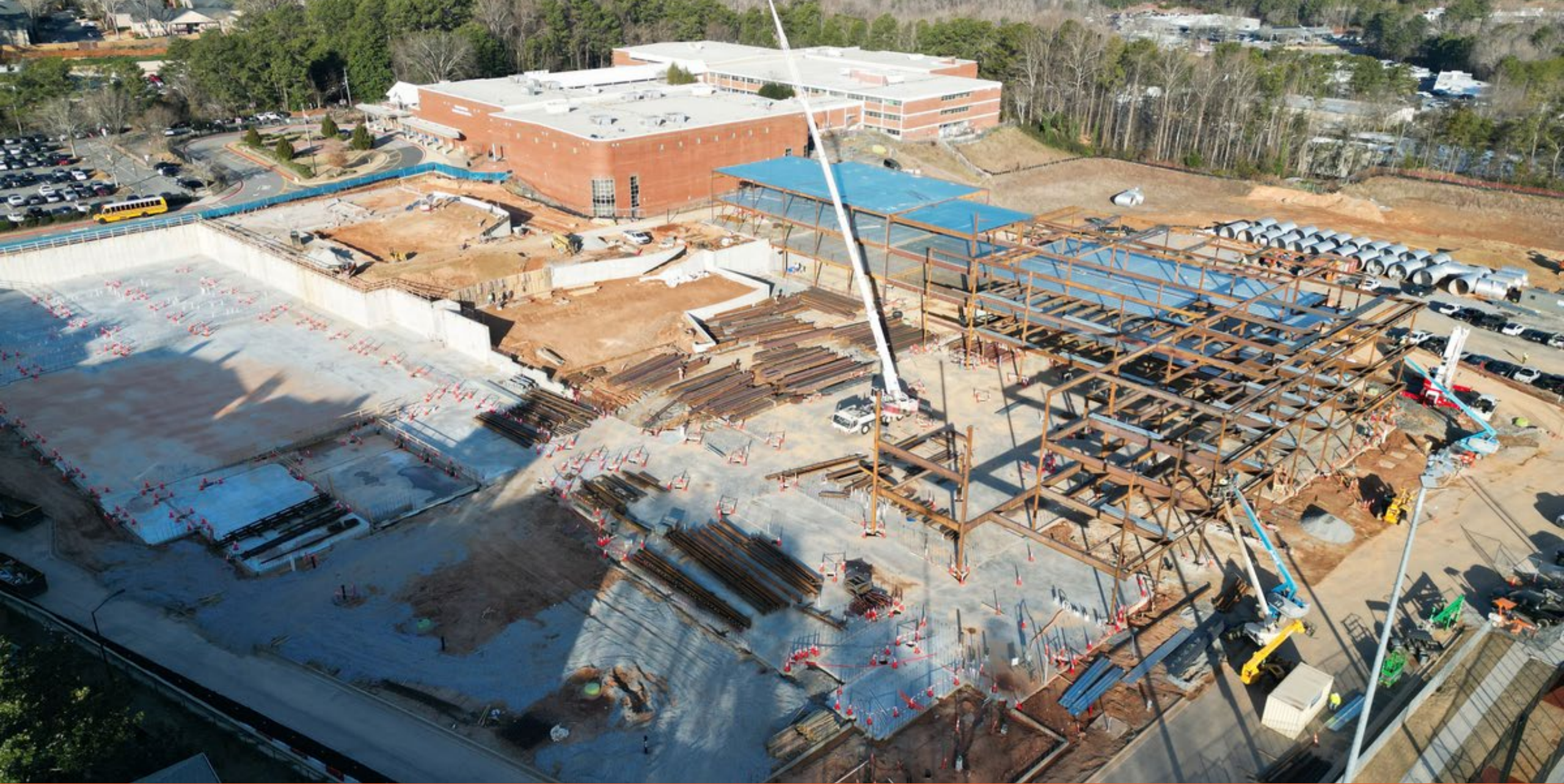
Main Building- Aerial view from South-East
