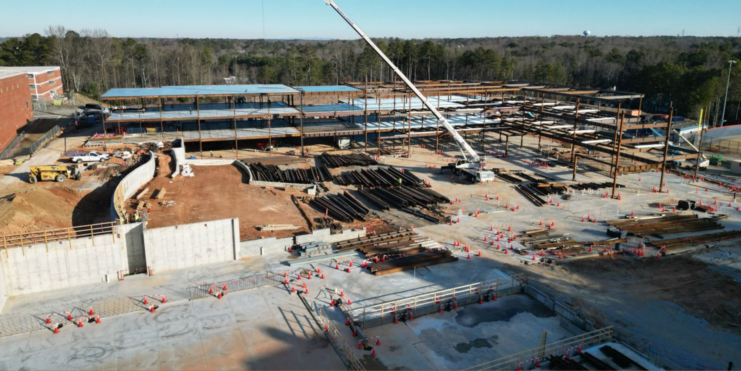
Aerial view- Steel Erection in progress.
