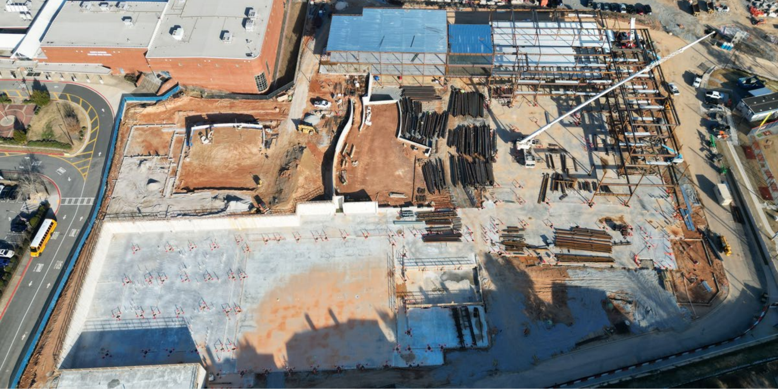
Site Progress Overview- Slab Pour, Foundation Walls and Steel Erection in progress.
