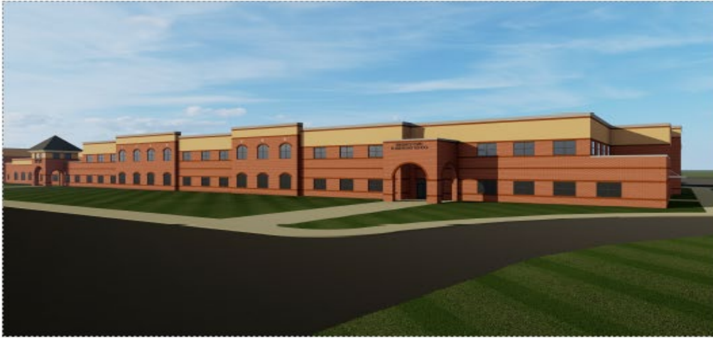
NORTH EXTERIOR - ELEMENTARY ENTRANCE
