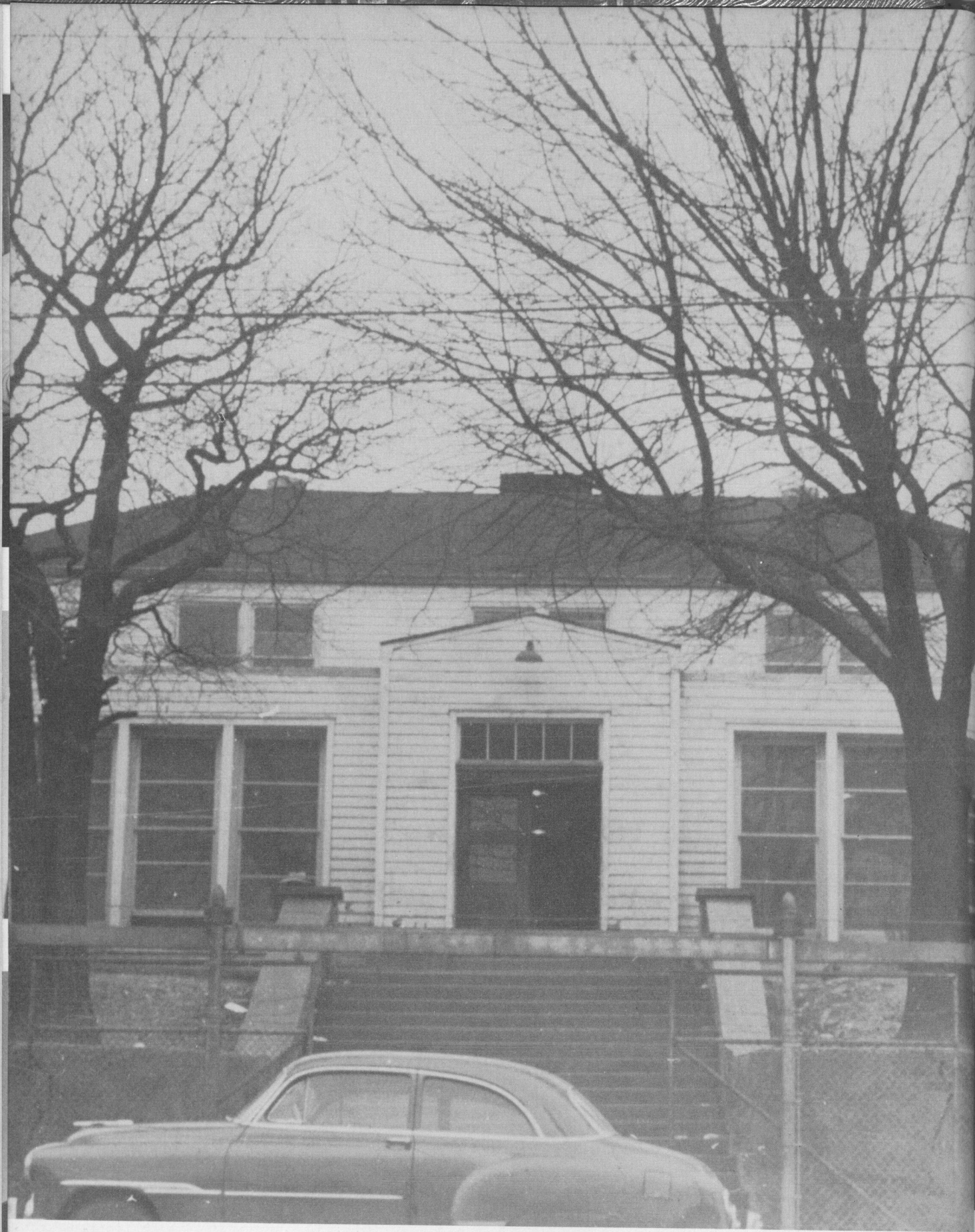
THE ACTIVITY BUILDING
