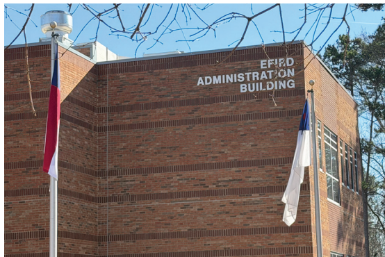
Efird Administration Building
