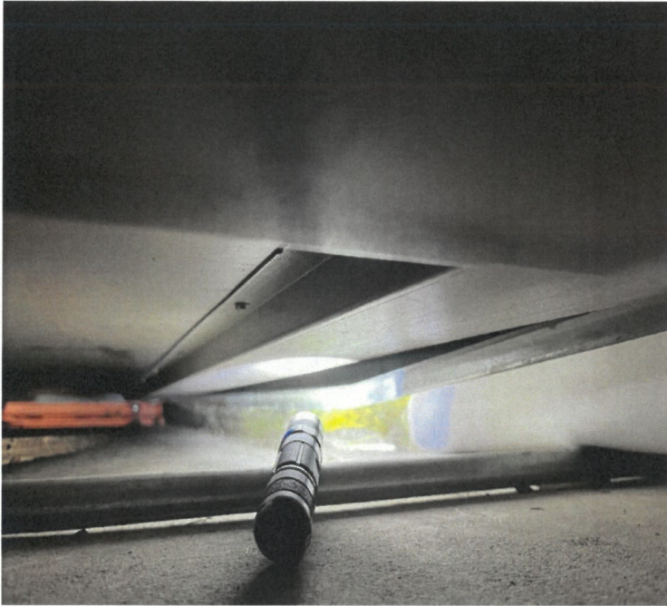
Collapsed Supply Duct (Above) Light from MER indicating leakage (below L&R)
