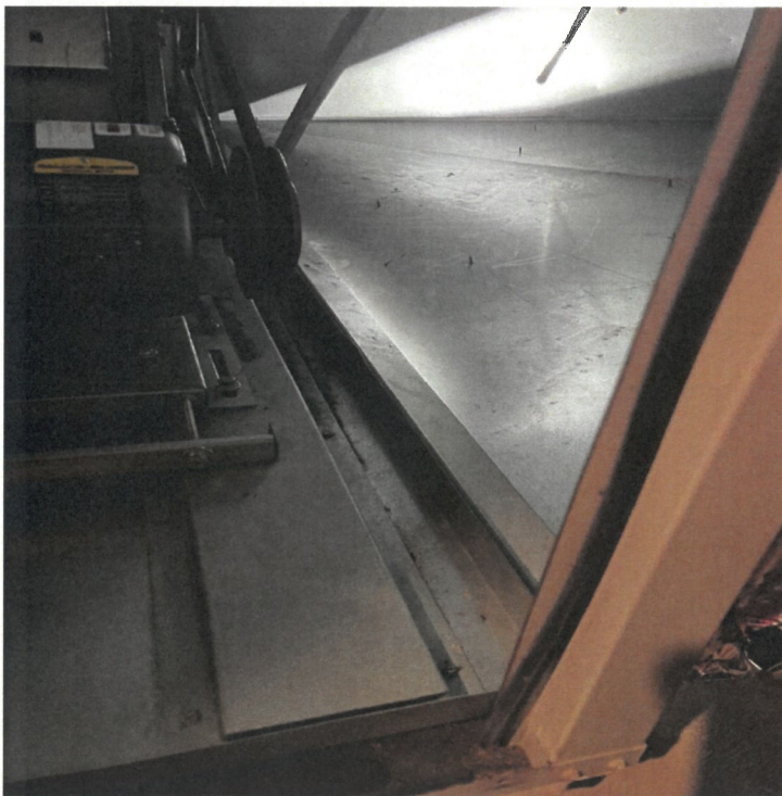
Collapsed Supply Duct (Above) Light from MER indicating leakage (below L&R)
