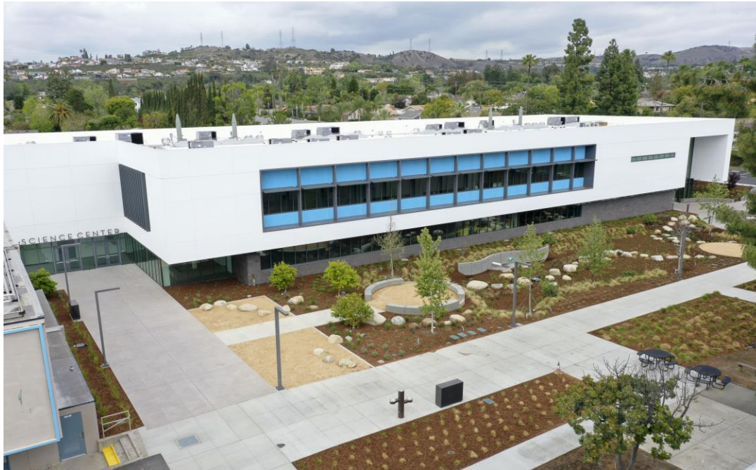
PHASE I: COMPLETED
