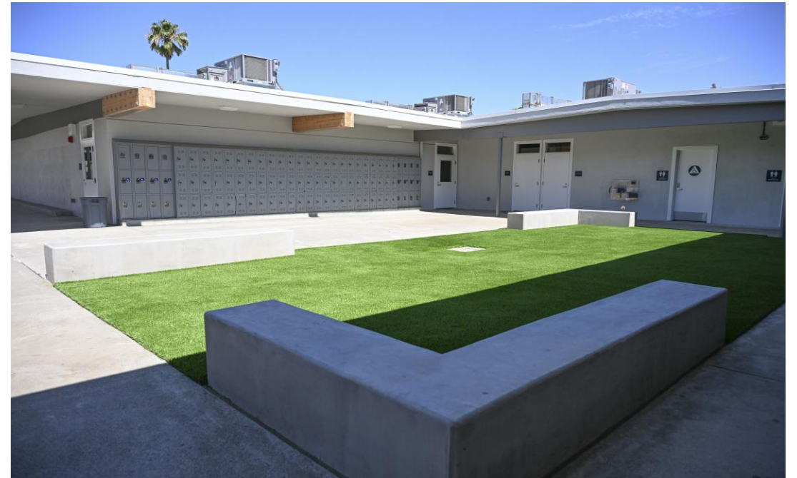
PHASE II: COMPLETED
