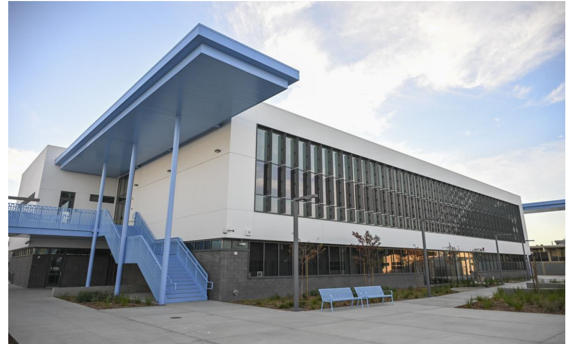
PHASE II: COMPLETED
