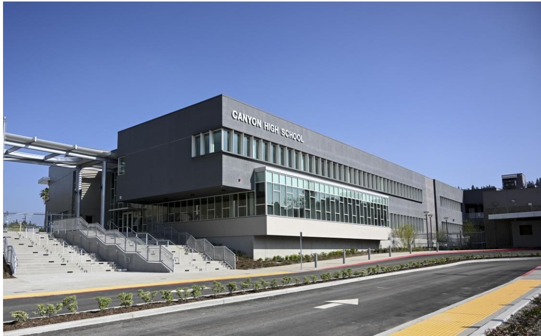
PHASE I: COMPLETED
