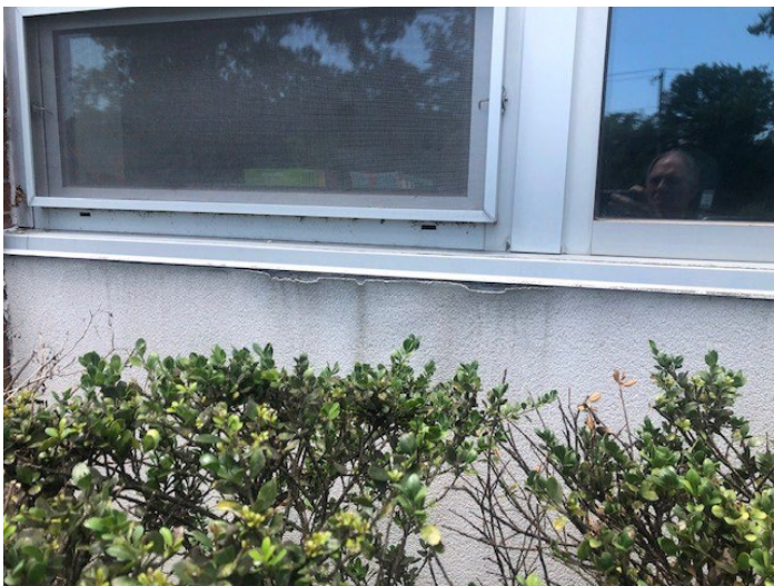
Typical lintel, caulking and EIFS repair conditions
