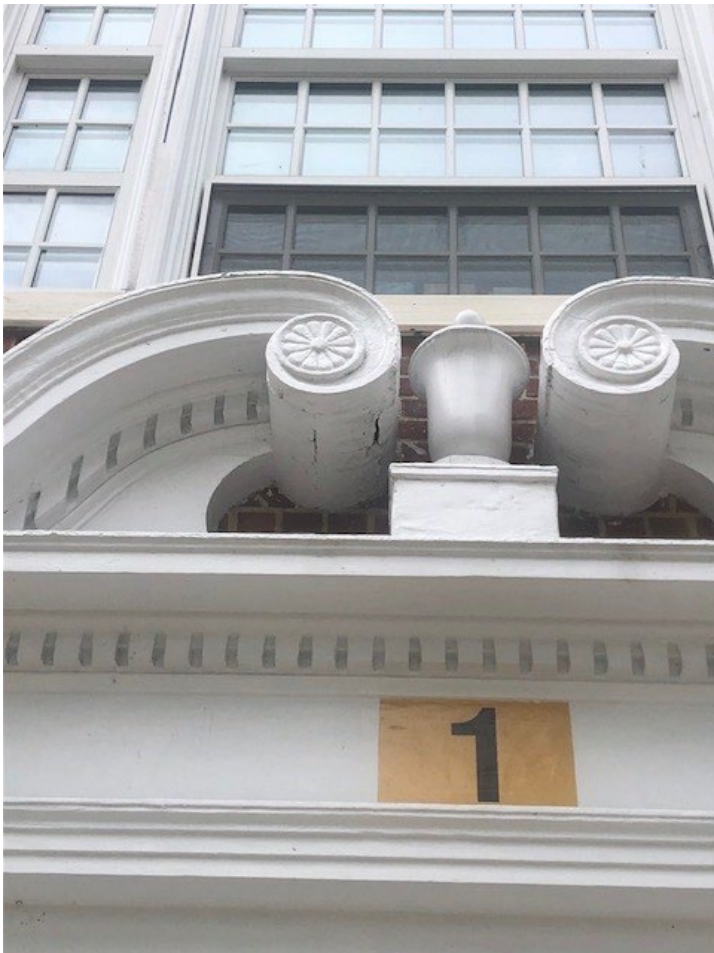
Typical sill and main entry header scroll repair conditions
