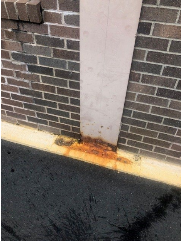
Typical steel base-at (13) locations
