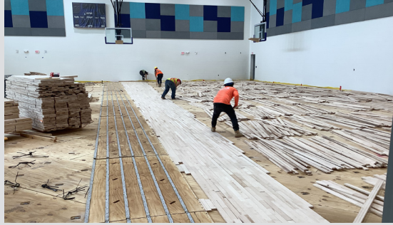
The wood strips must sit in a controlled environment for 7 days before it can be installed.
