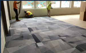
First floor tile install and rolling (Area B)
