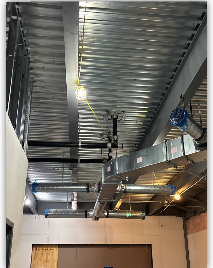
Above Ceiling MEPs + Drywall in UPK Addition
