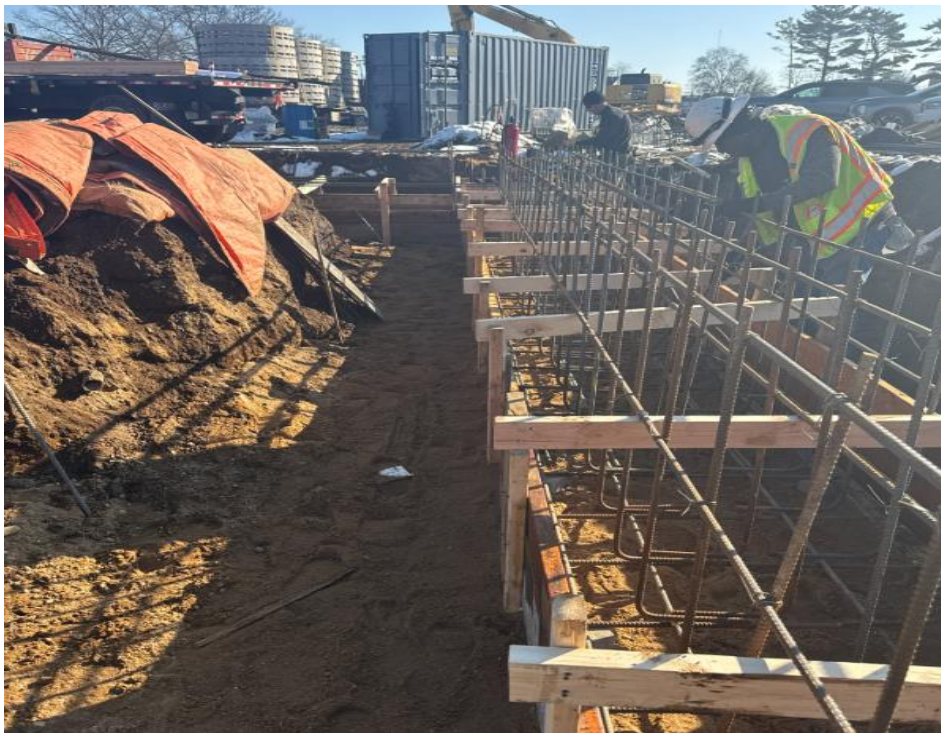
Hempstead ABGS MS – Footings & Foundation wall Rebar
