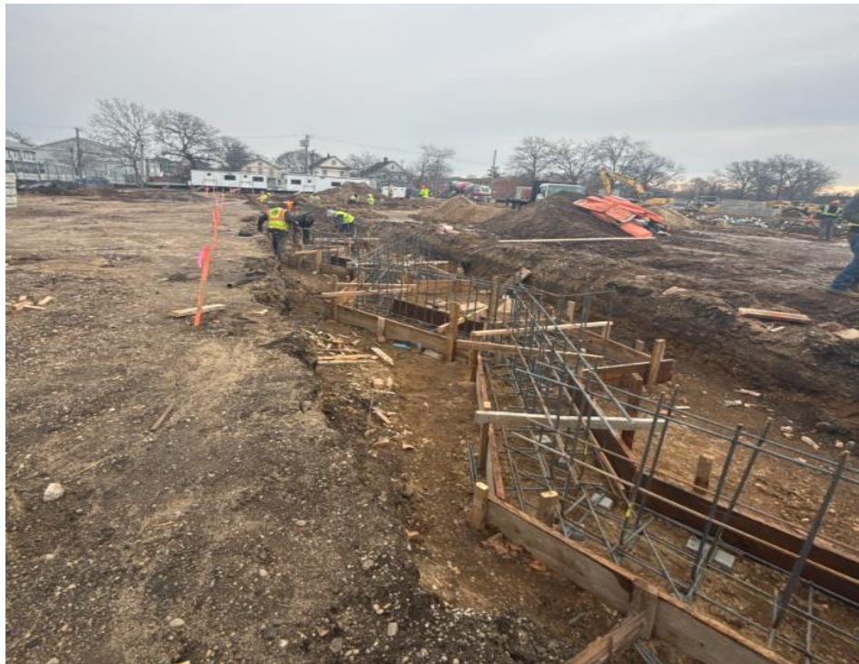
Hempstead ABGS MS – Footings & Foundation wall Rebar
