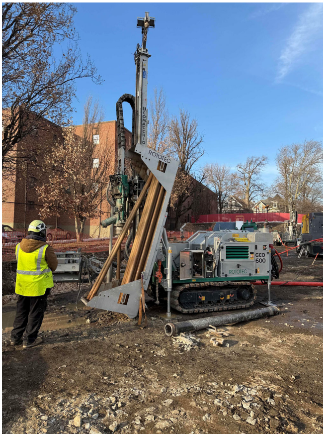
Geothermal drilling rig, December 17
