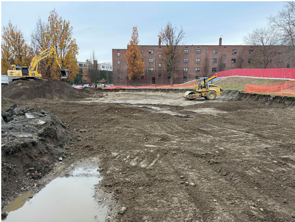
Pierce Park excavation underway, December 04
