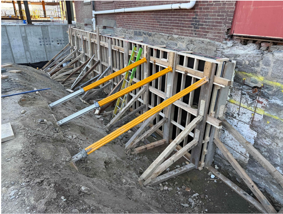
Historic Building, foundation work, December 11
