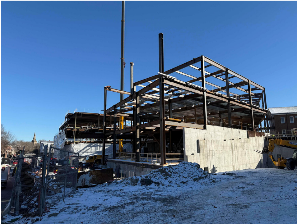
Building structure, December 15
