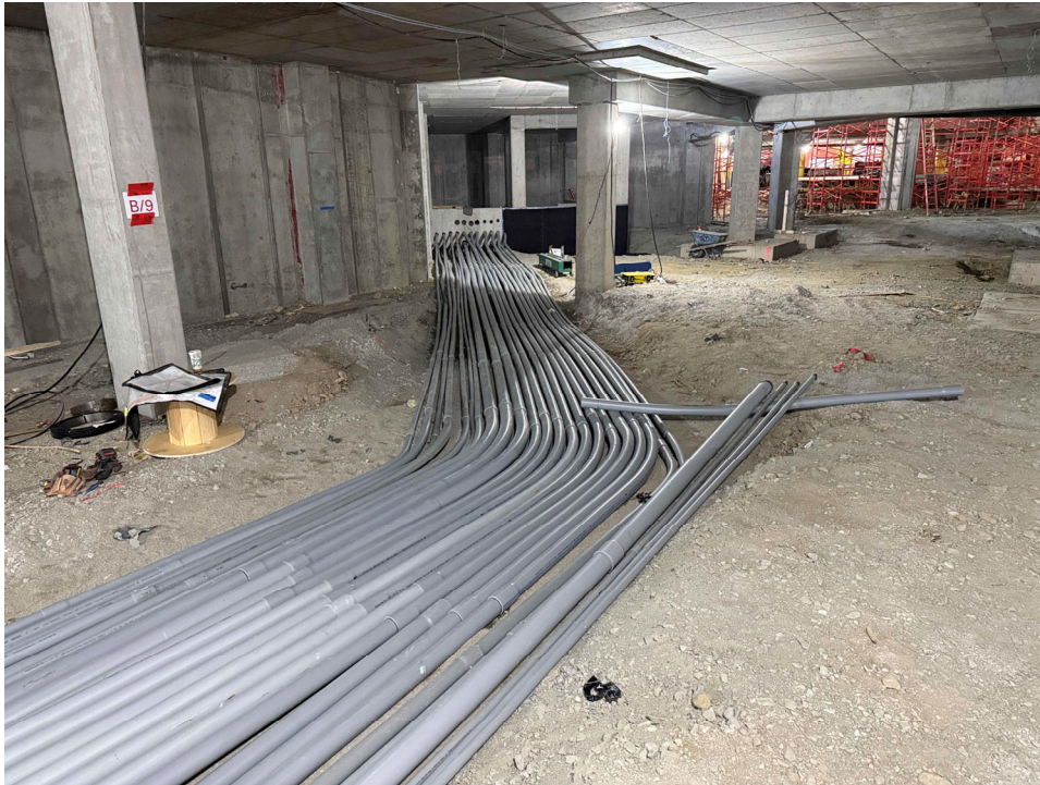
Underground conduit, Building A garage level, December 15
