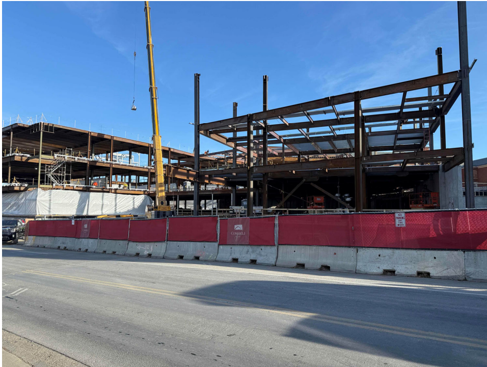
Building structure, December 09
