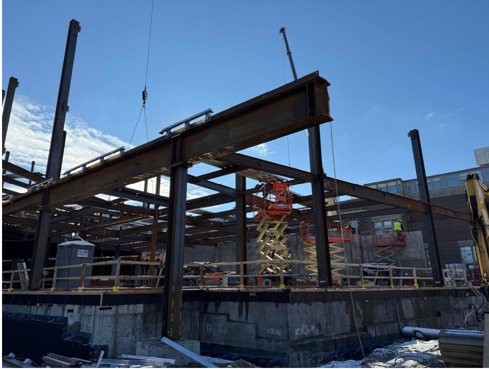
Building B steel structure, December 03
