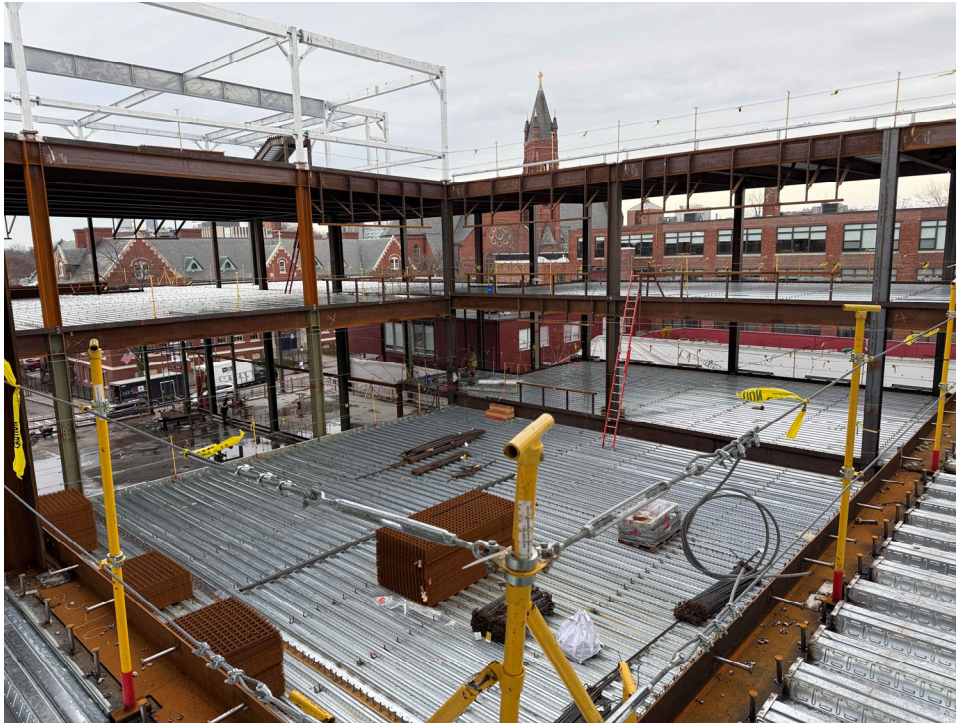
Building A steel structure, December 04
