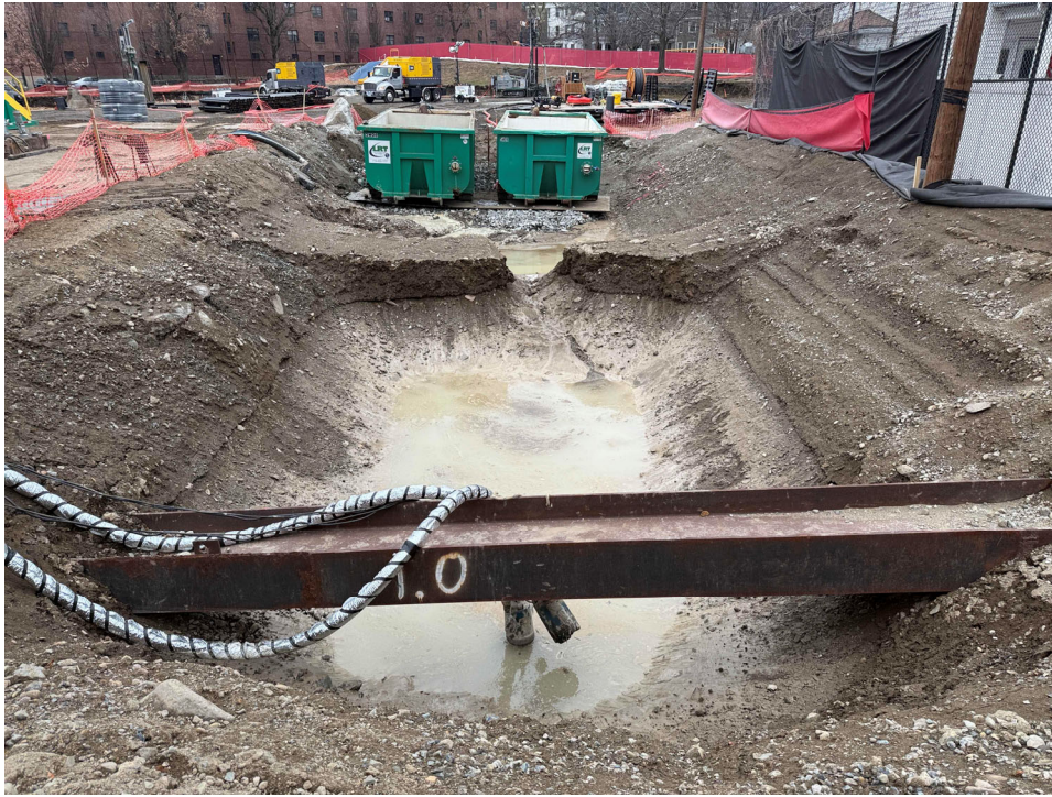
Water management for geothermal drilling, December 23
