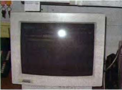
Operating Control Location
