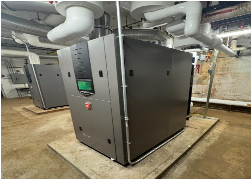
Hempstead McNeil ES – Boiler replacement
