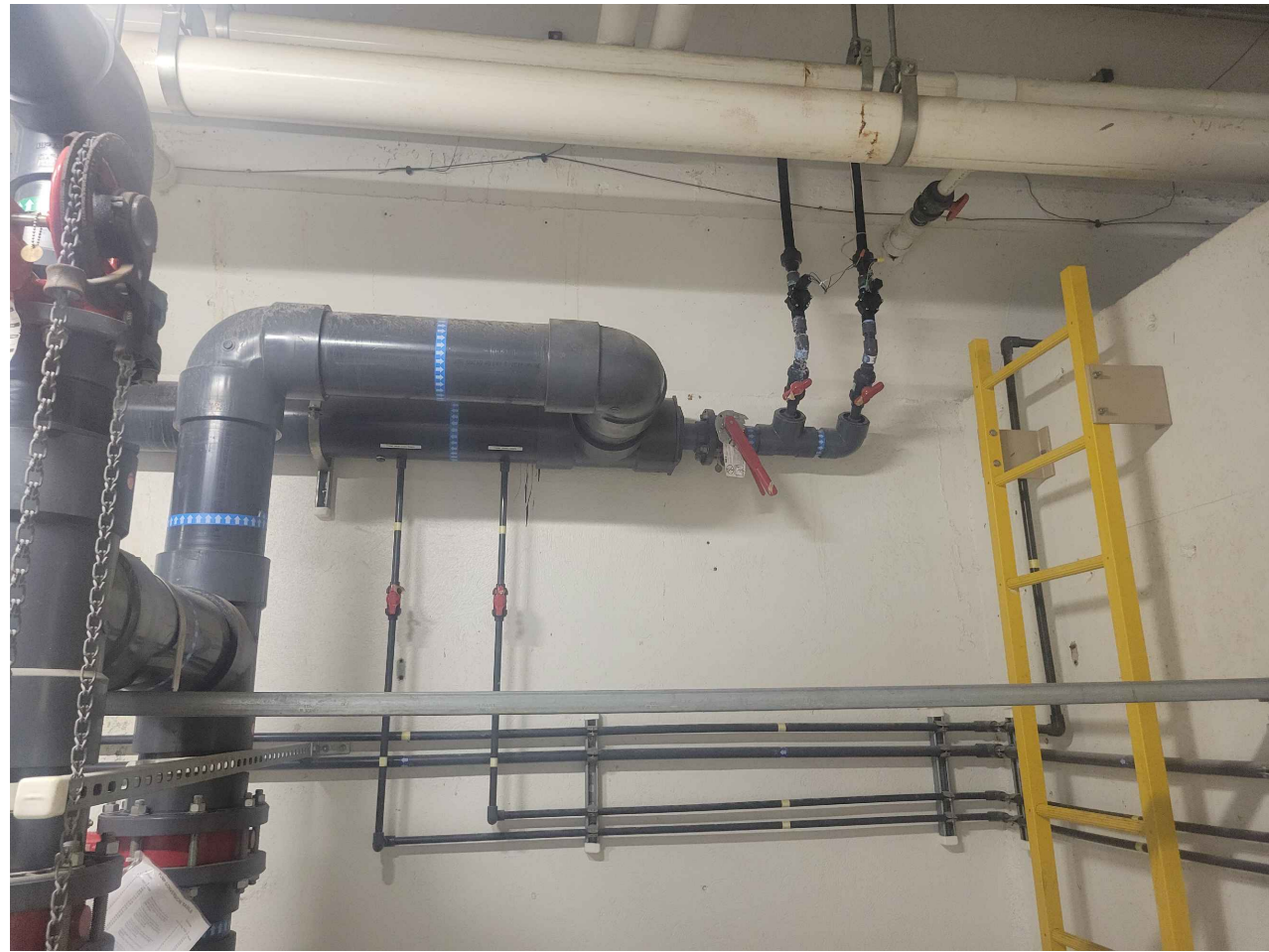
10 AQ0.2 EXISTING CHEMICAL INJECTIONS NTS
