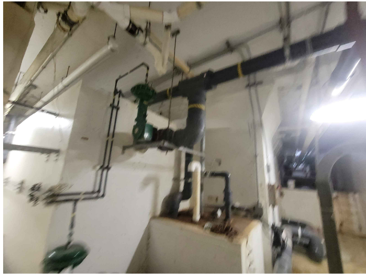
9 AQ0.2 EXISTING GUTTER FISHER VALVE NTS
