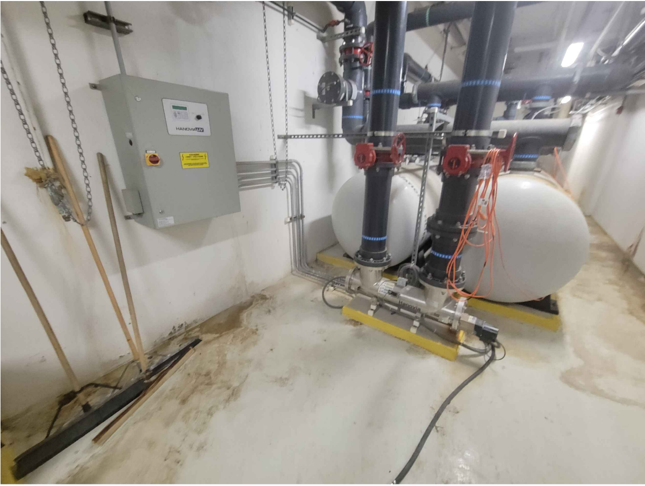
7 AQ0.2 EXISTING UV CHAMBER & CABINET NTS
