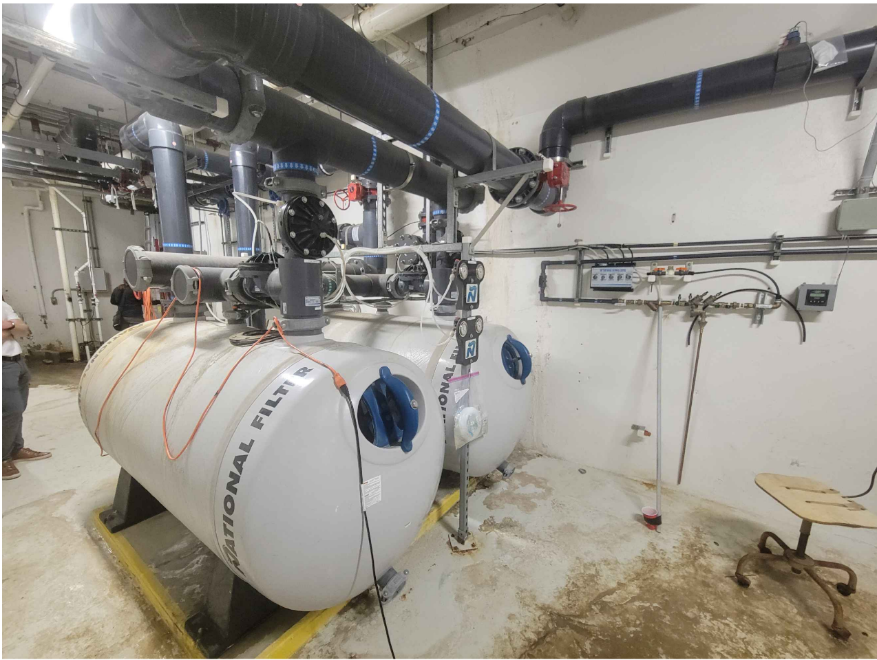
3 AQ0.2 EXISTING SAND FILTERS NTS
