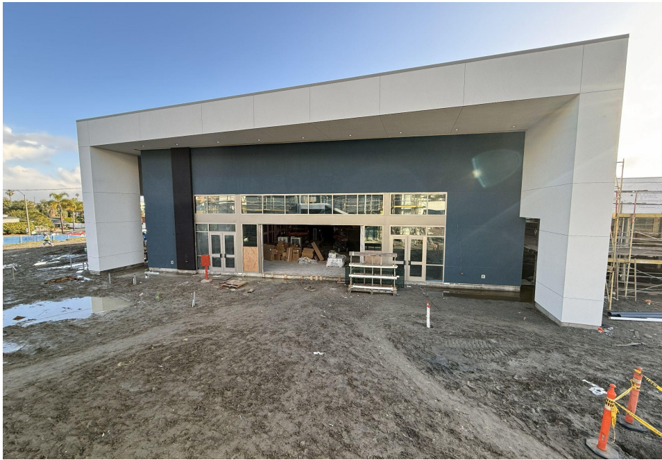
Bldg B MPR Door and Window Installation
