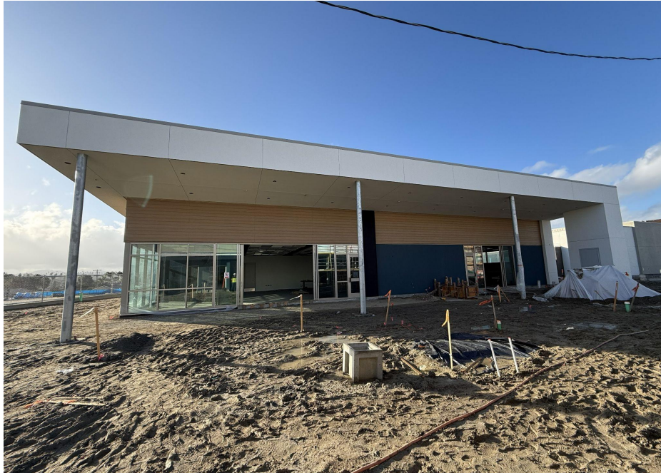
Bldg C North - Library & STEAM
