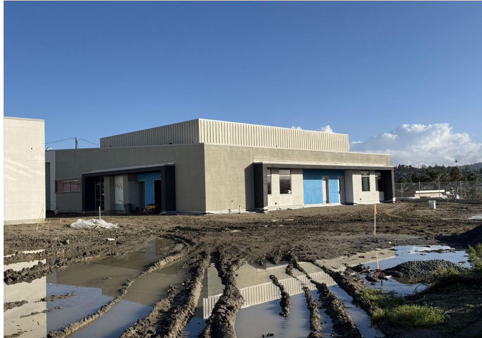
Bldg C South Exterior Paint
