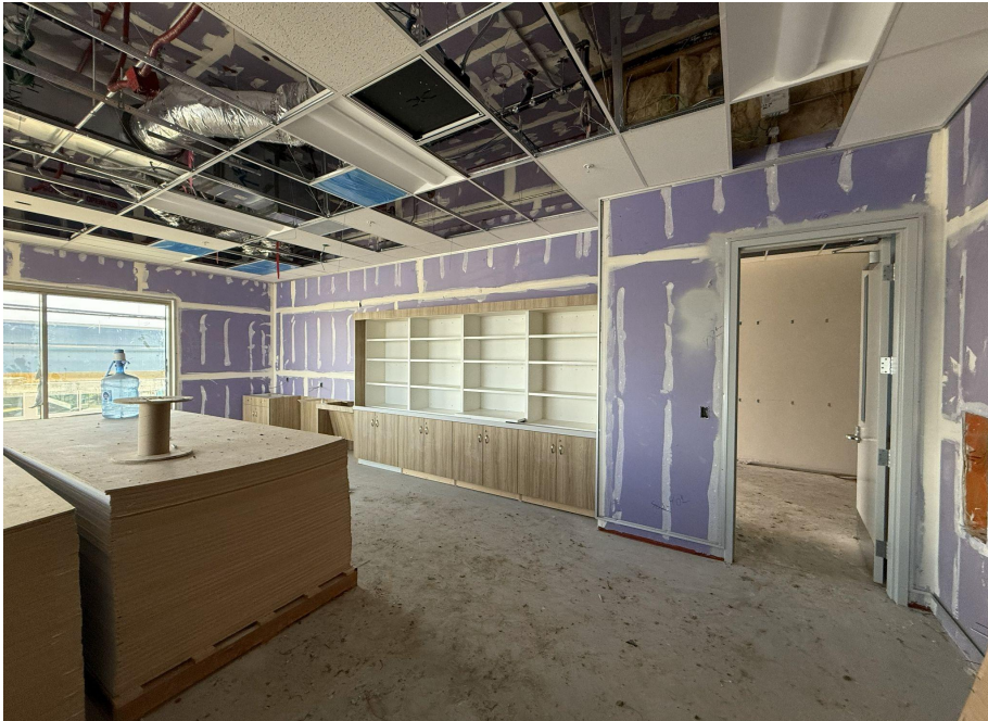
Bldg A 2nd Floor Classroom Casework Installation
