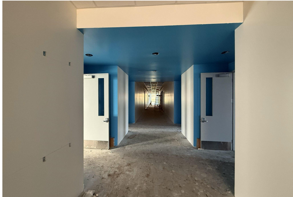
Bldg A 2nd Floor Corridor Doors and Paint
