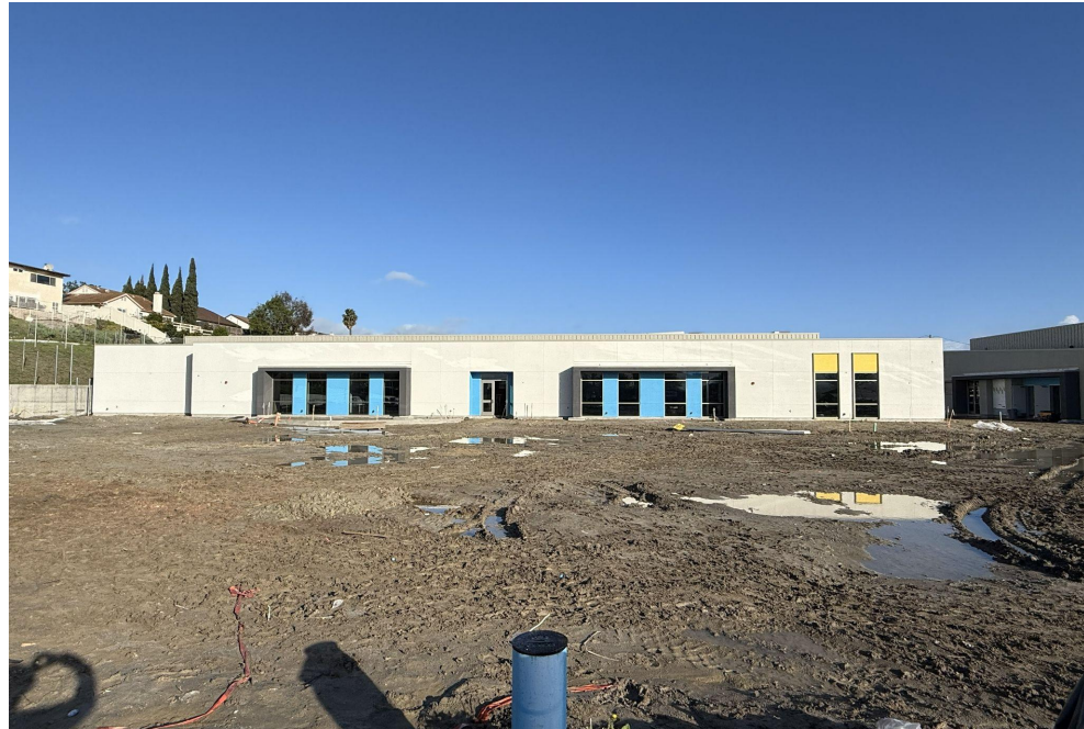
Bldg A South Exterior Paint
