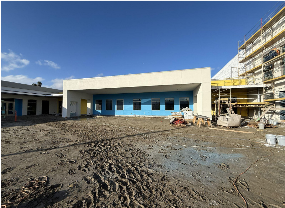
Bldg A West Paint (Kinder Classrooms)
