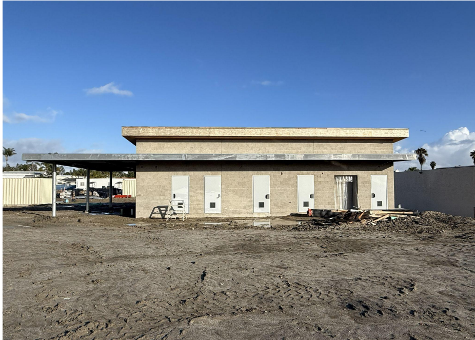
Bldg D Exterior Doors and Canopy Roof Installation
