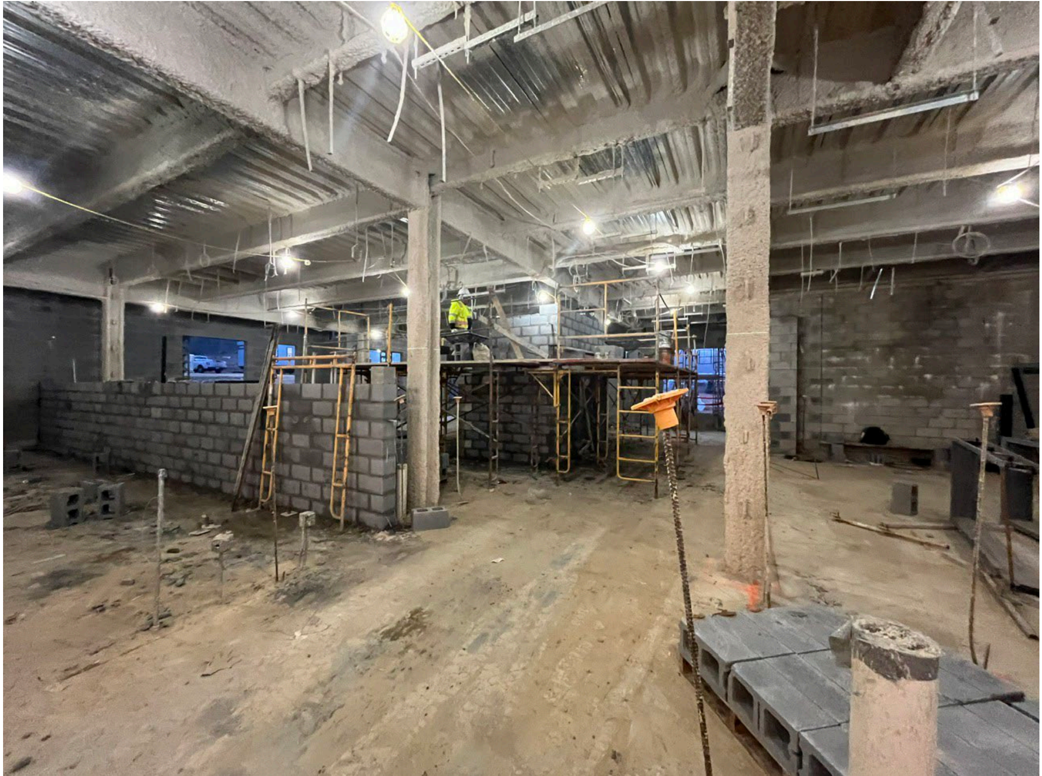
NORTH EAST MIDDLE / HIGH SCHOOL – REPLACEMENT – CLASSROOMS
