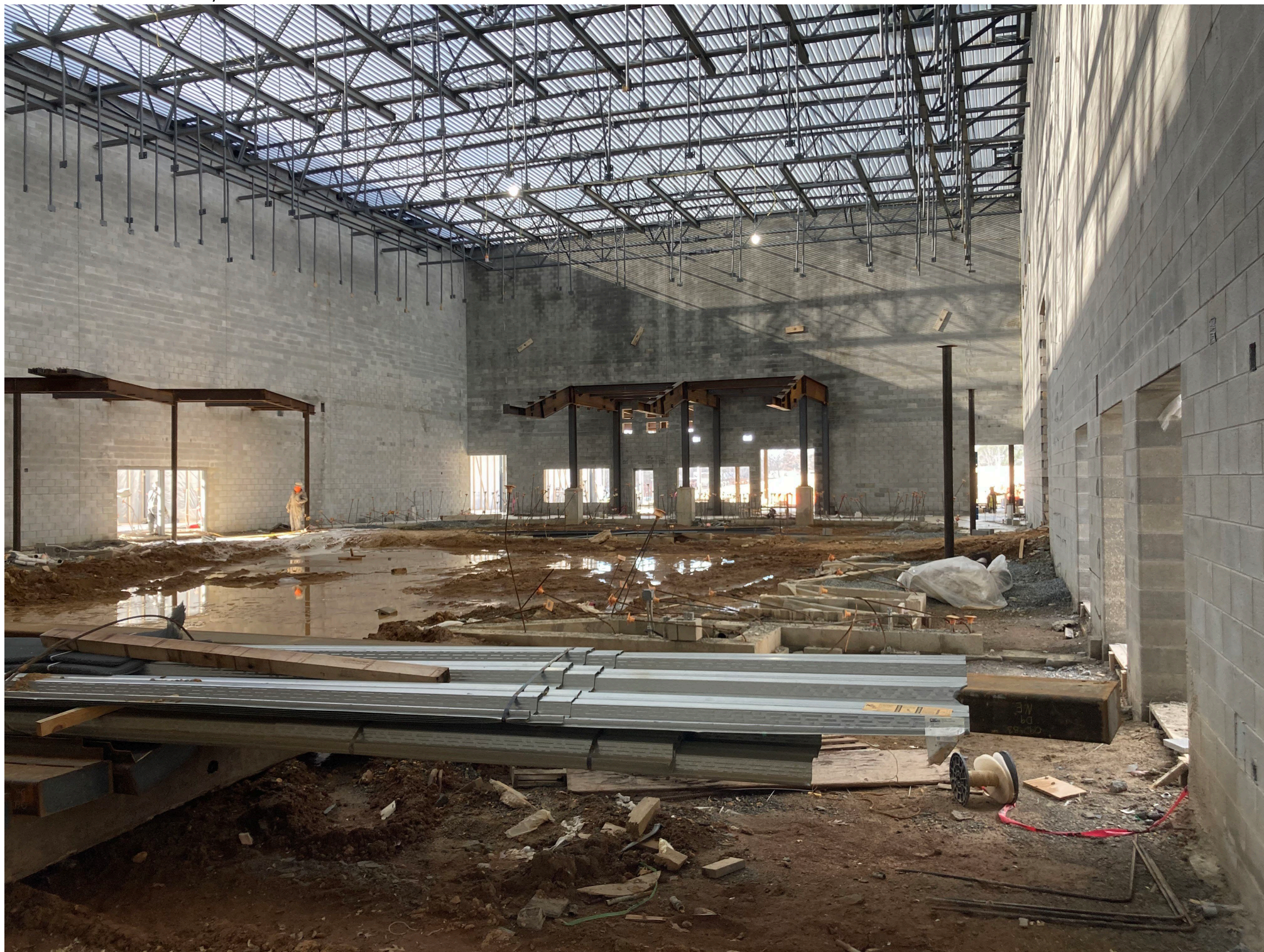
NORTH EAST MIDDLE / HIGH SCHOOL – REPLACEMENT – AUDITORIUM
