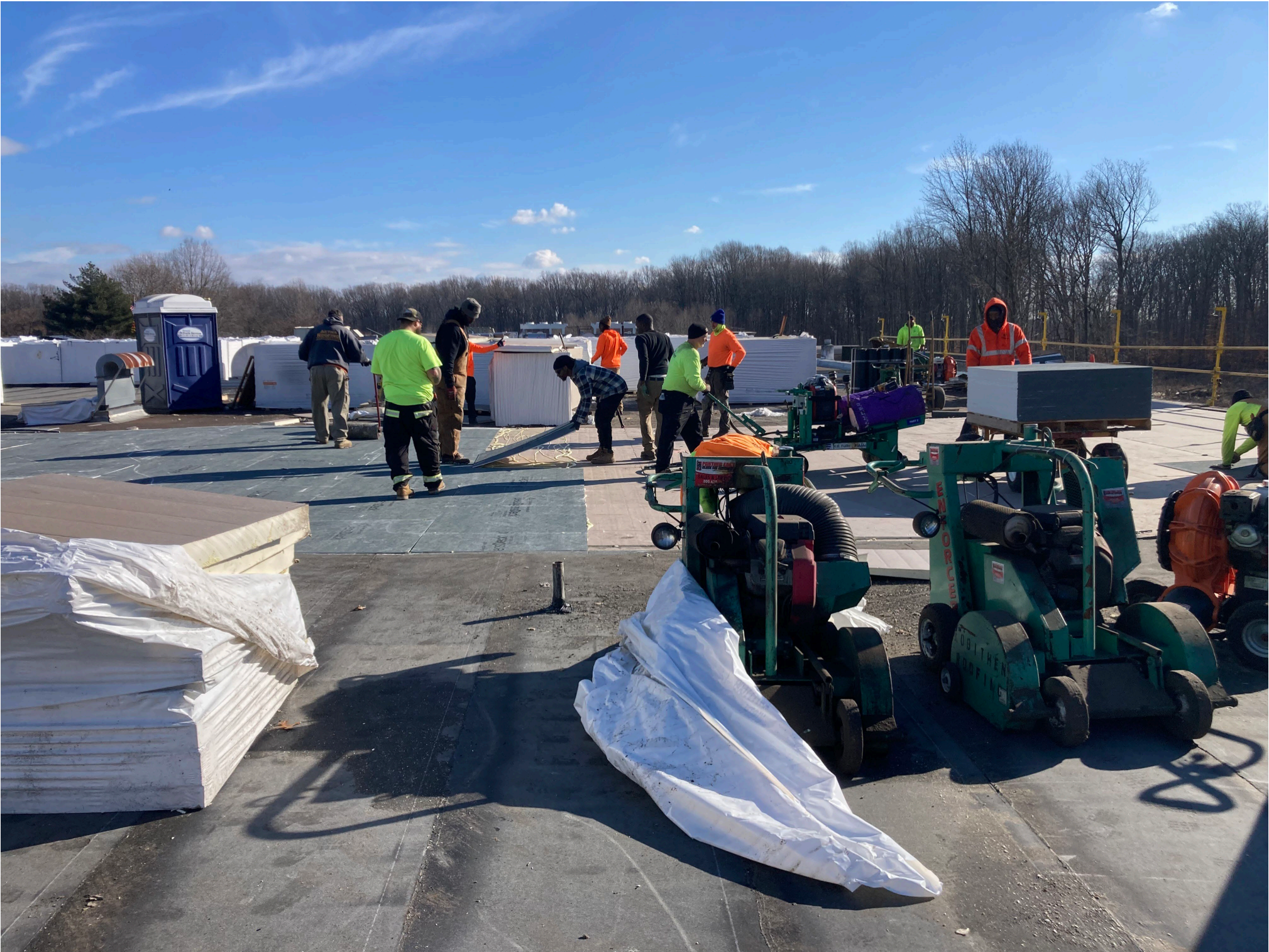
ADMINISTRATIVE SERVICES CENTER – ROOF REPLACEMENT
