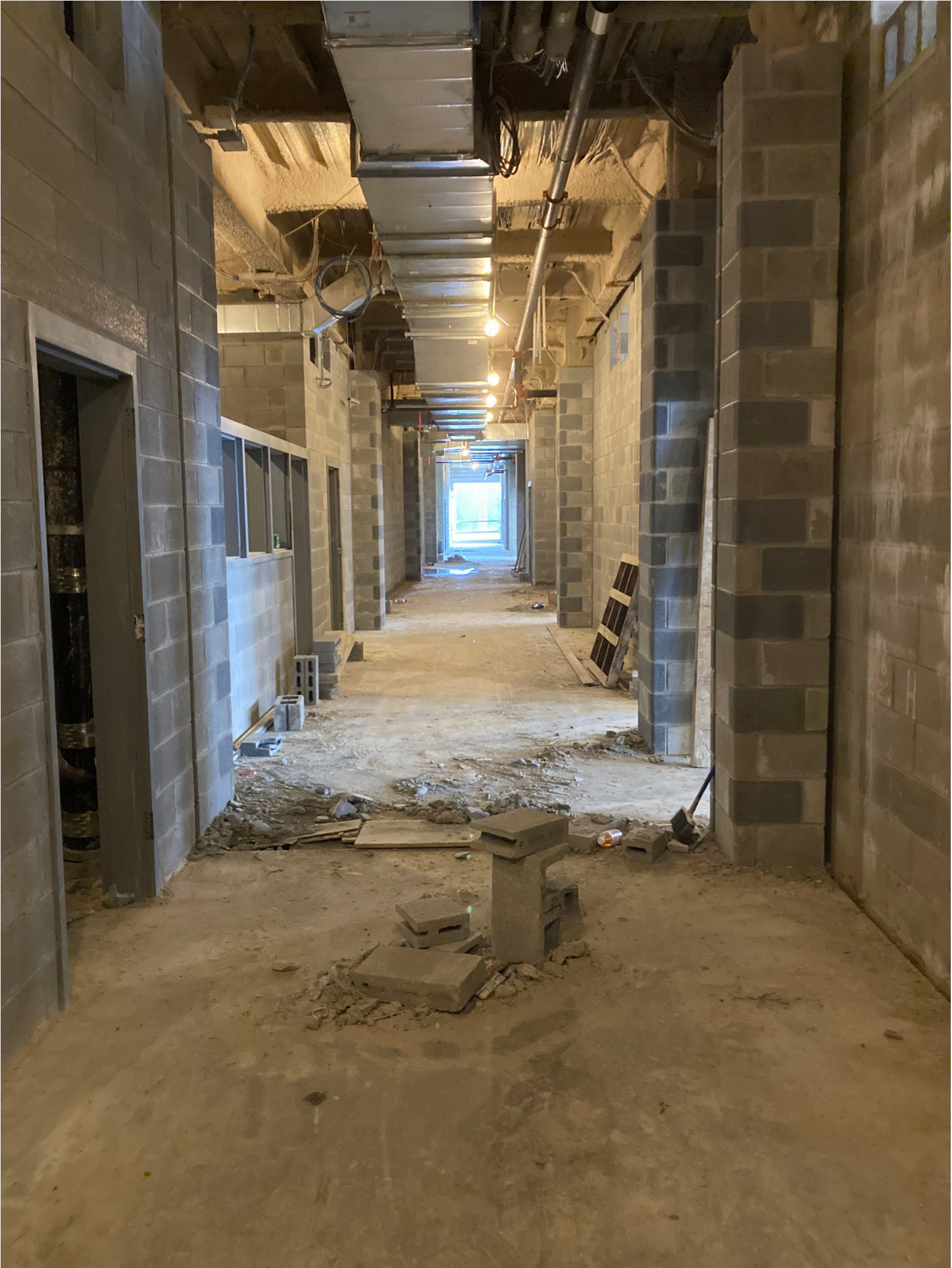
NORTH EAST MIDDLE / HIGH SCHOOL – REPLACEMENT – CLASSROOM HALLWAY
