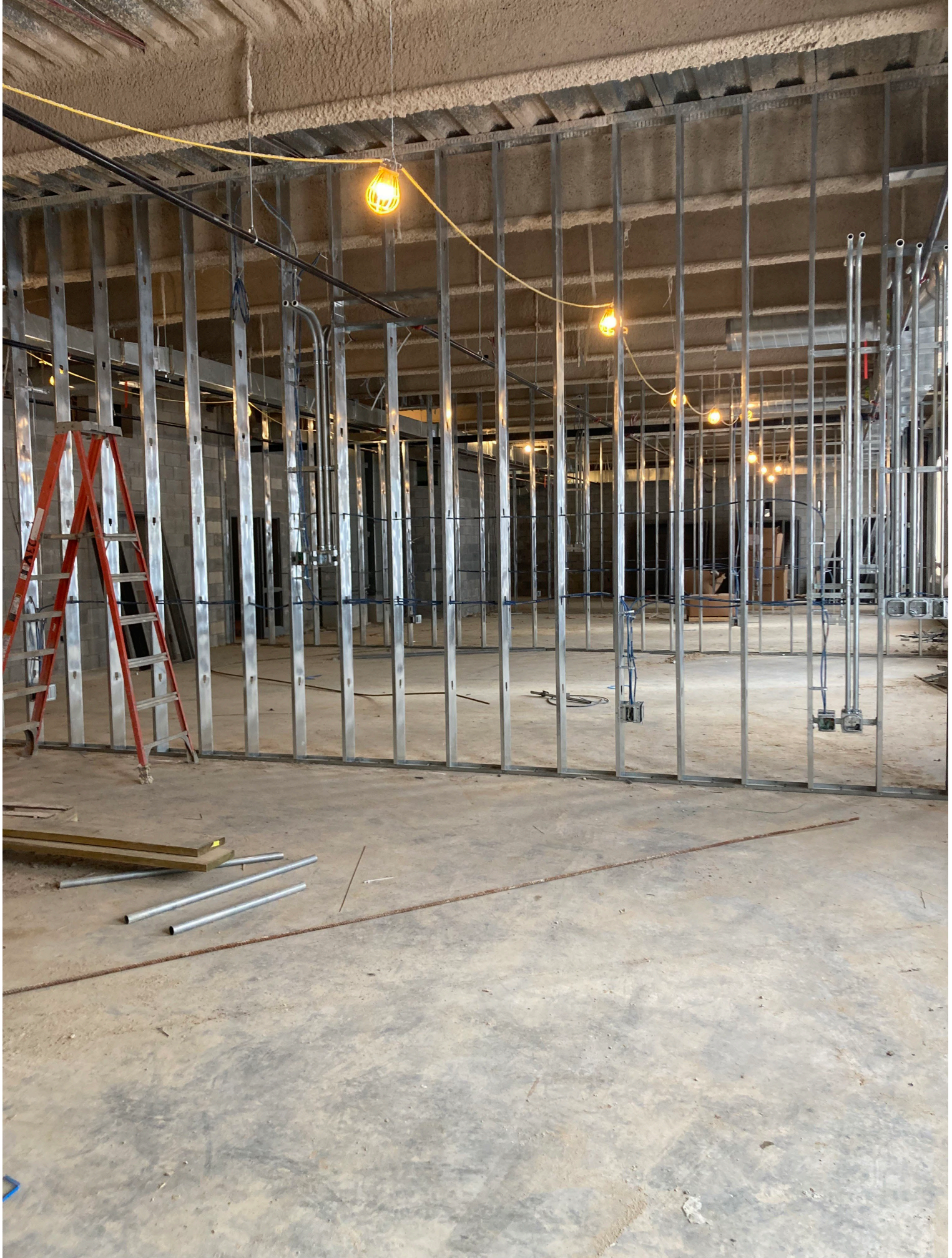
NORTH EAST MIDDLE / HIGH SCHOOL – REPLACEMENT – CLASSROOMS
