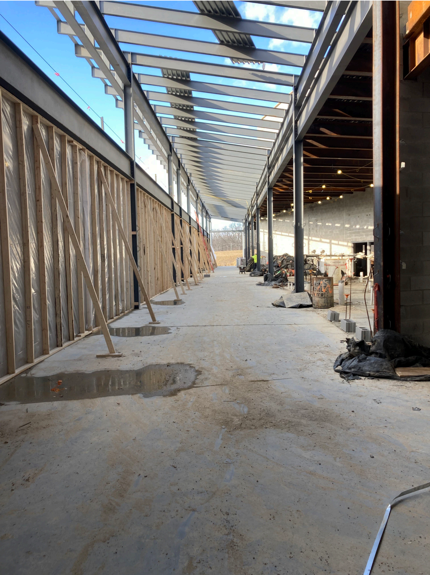
NORTH EAST MIDDLE / HIGH SCHOOL – REPLACEMENT – MAIN “BOARDWALK” CORRIDOR
