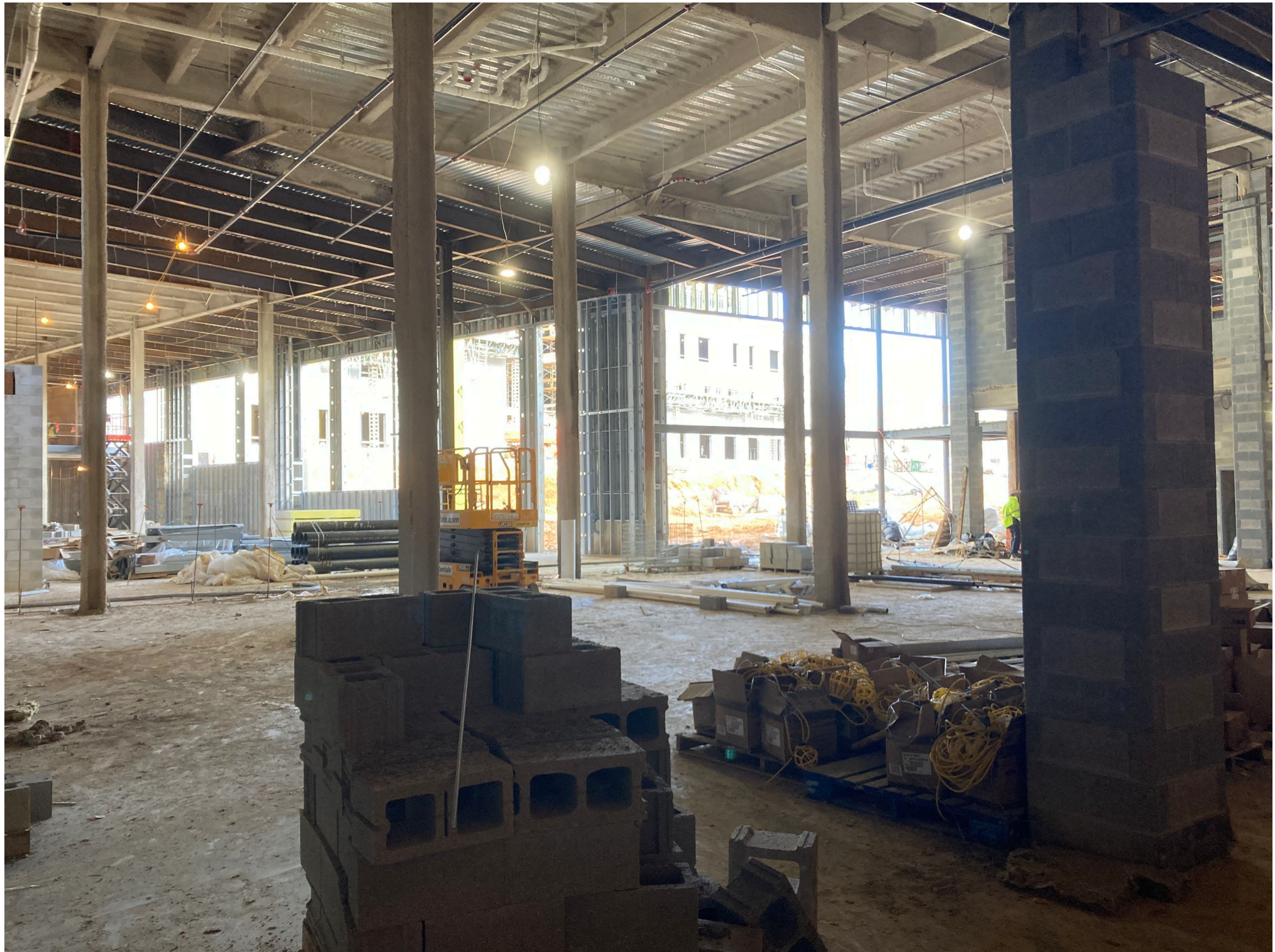
NORTH EAST MIDDLE / HIGH SCHOOL – REPLACEMENT – MIDDLE SCHOOL CAFETERIA
