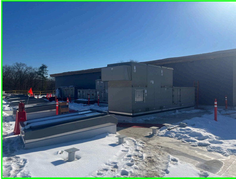
Photo 1: delivery and placement of mechanical rooftop equipment and skylights
