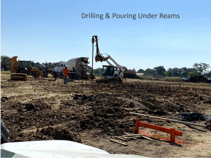
Wire Cages for Under Reams
