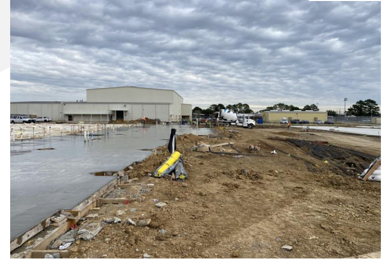
Grade Beams and Plumbing Rough-In
