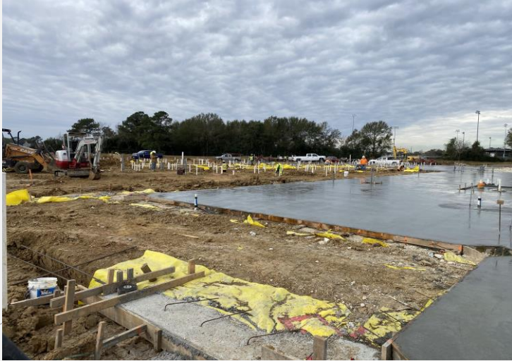
Entry Drive Concrete
