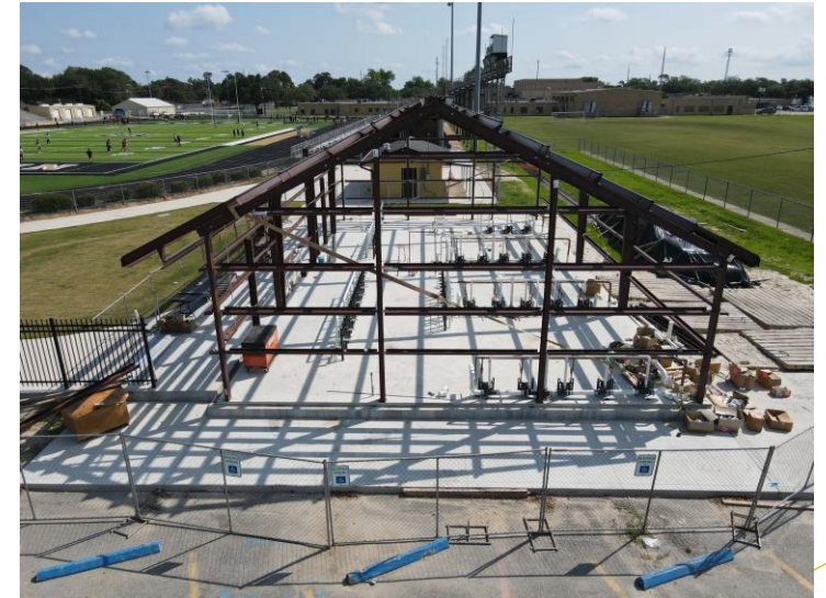
Home Side Restroom
