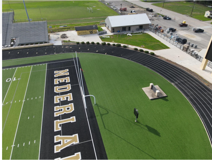
Home Side Restroom
