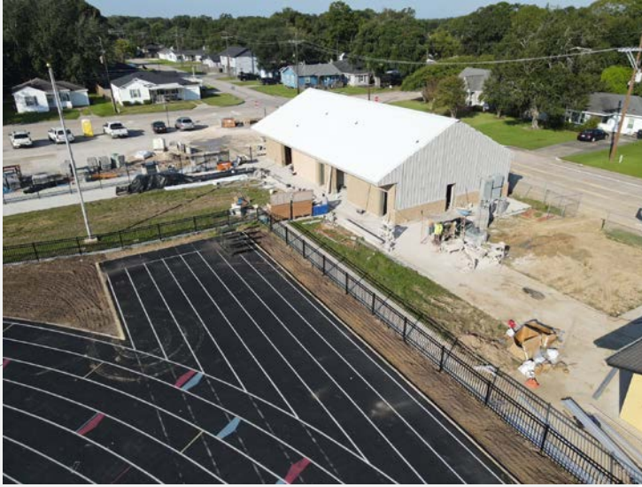
Visitor Side Restroom
