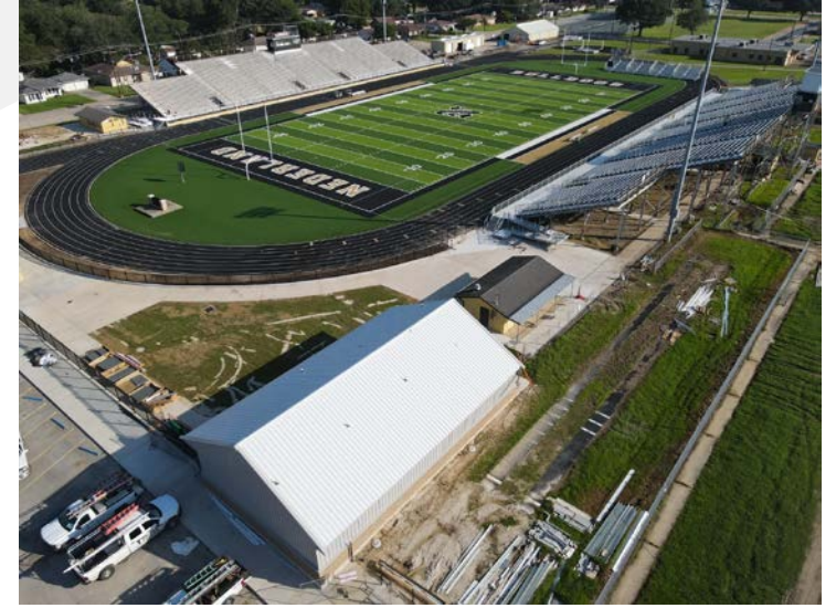
Home Side Restroom
