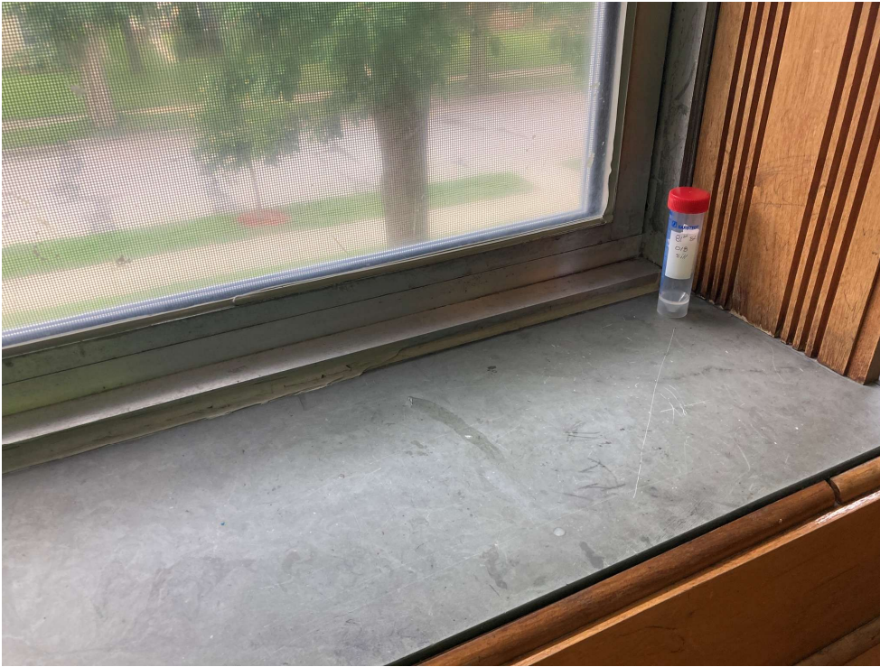
Figure 1: Example of a sill within one of the classrooms
