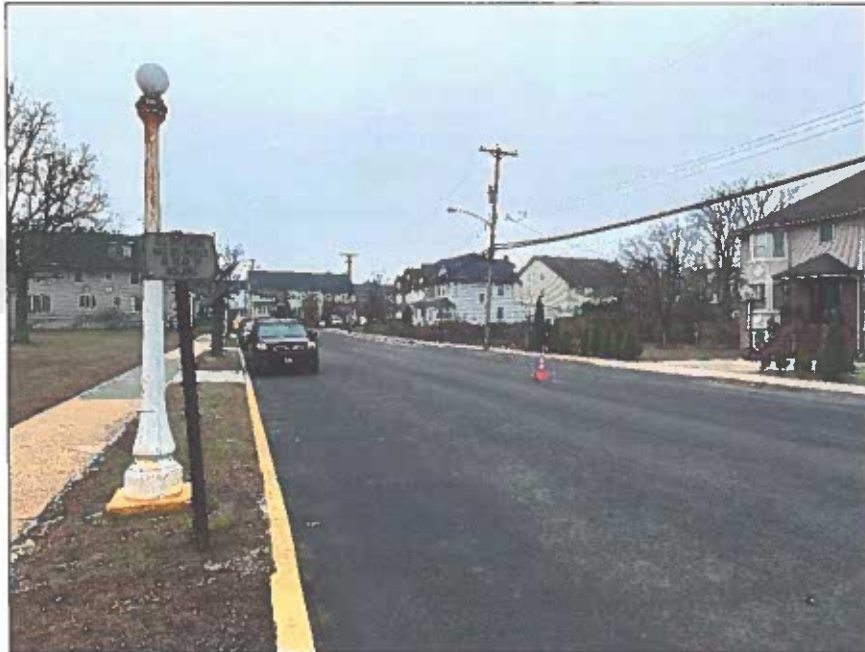
Manetta Avenue Street Scene View: South
