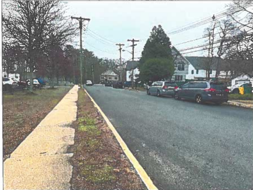
Linden Avenue Street Scene View: East
