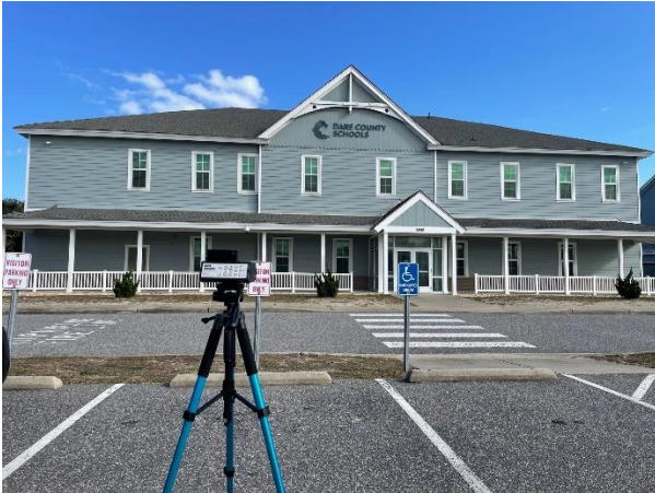
Dare County Schools Administrative Offices – Front exterior
