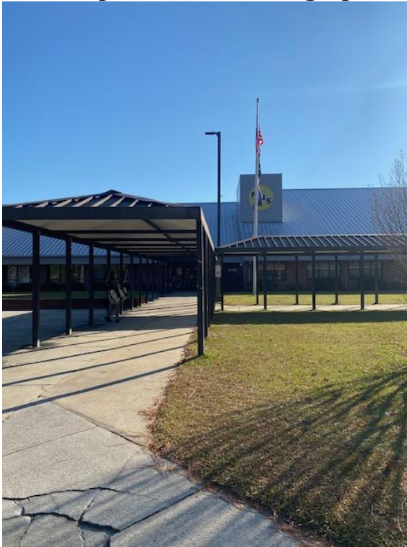
Manteo High School – Front Exterior
