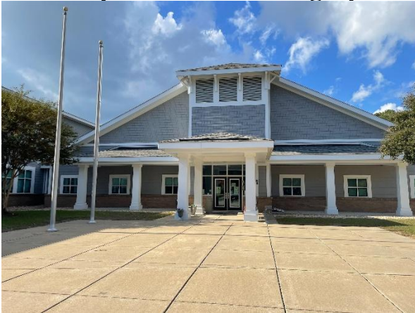
Manteo Middle School – Front Exterior
