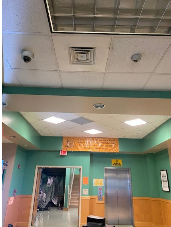
Main Entrance Hall
