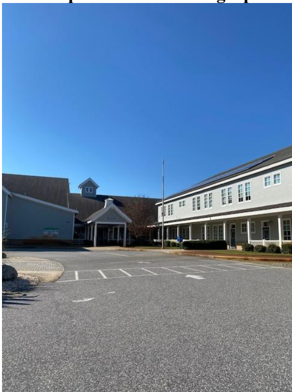
Cape Hatteras Elementary – Front exterior
