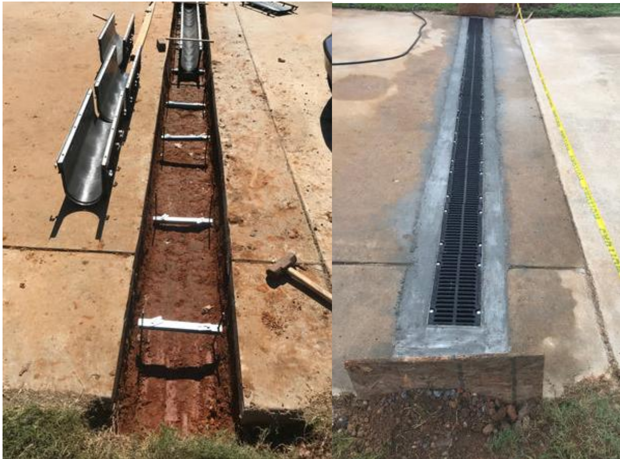
Edge drain during construction and at completion
