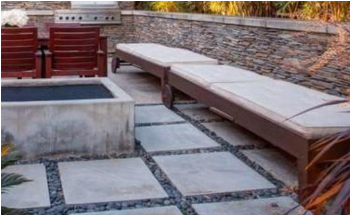
Example of concrete panels with drain rock
