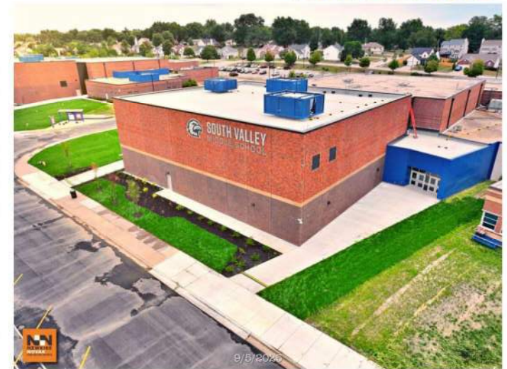
SVMS Exterior View
