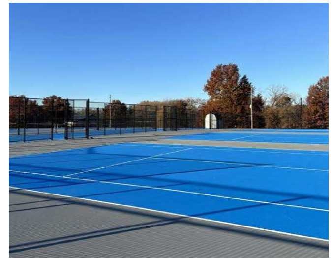
North Courts Looking Southwest
