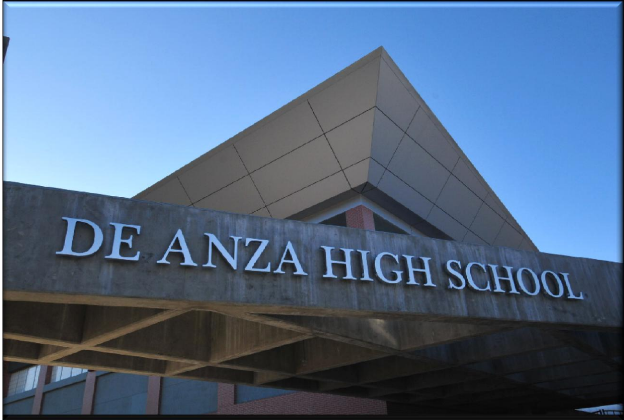
De Anza High School Replacement Campus (3521208-01)
