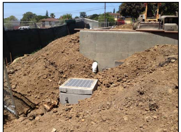
Storm drain connection
