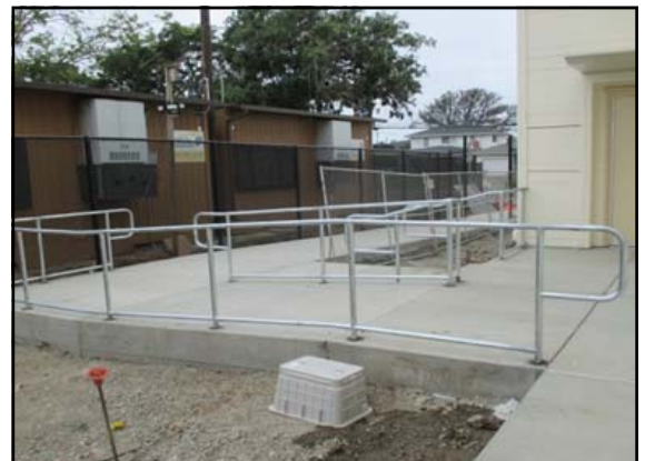
New handrails ADA ramp at south side of the building
