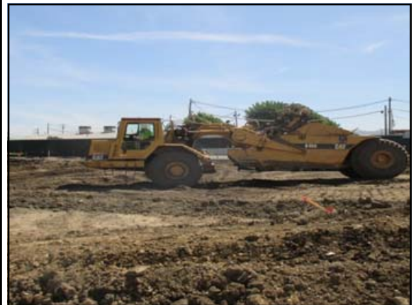
Site Grading for future playground area
