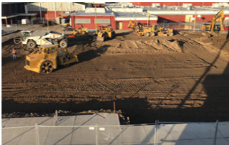
Richmond HS - Soil Compaction for Gym Pad
