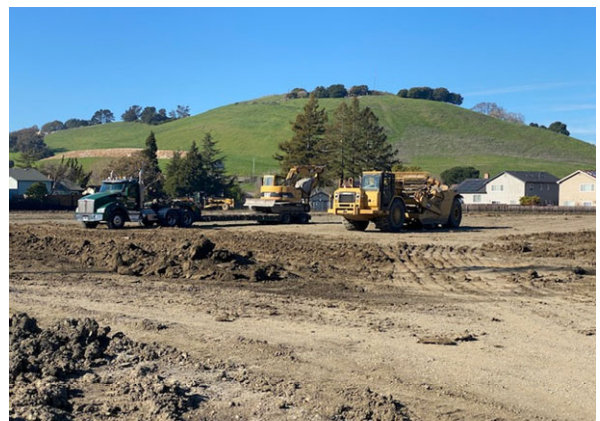
Grading and preparation for lime treat at the baseball fields
