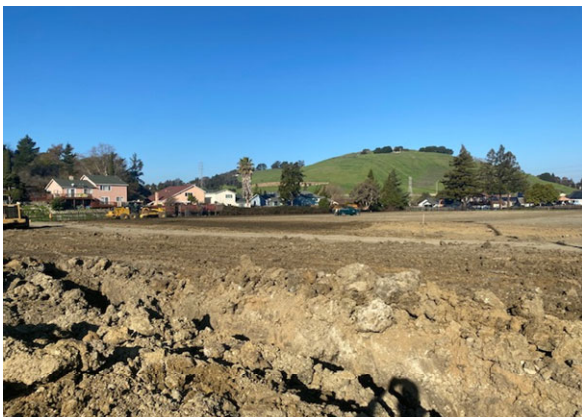
Final removal of interim campus utilities demo
