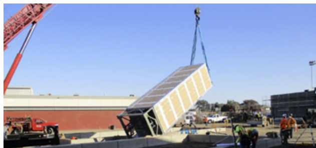
Richmond HS - Installing Science Building Elevator
