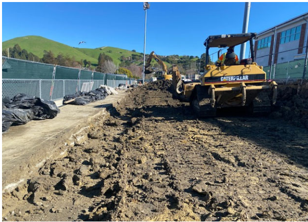
Grading work for new bleacher area
