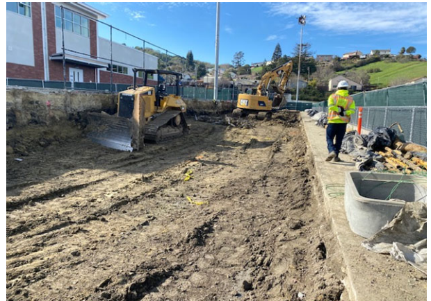
Grading work for new bleacher area
