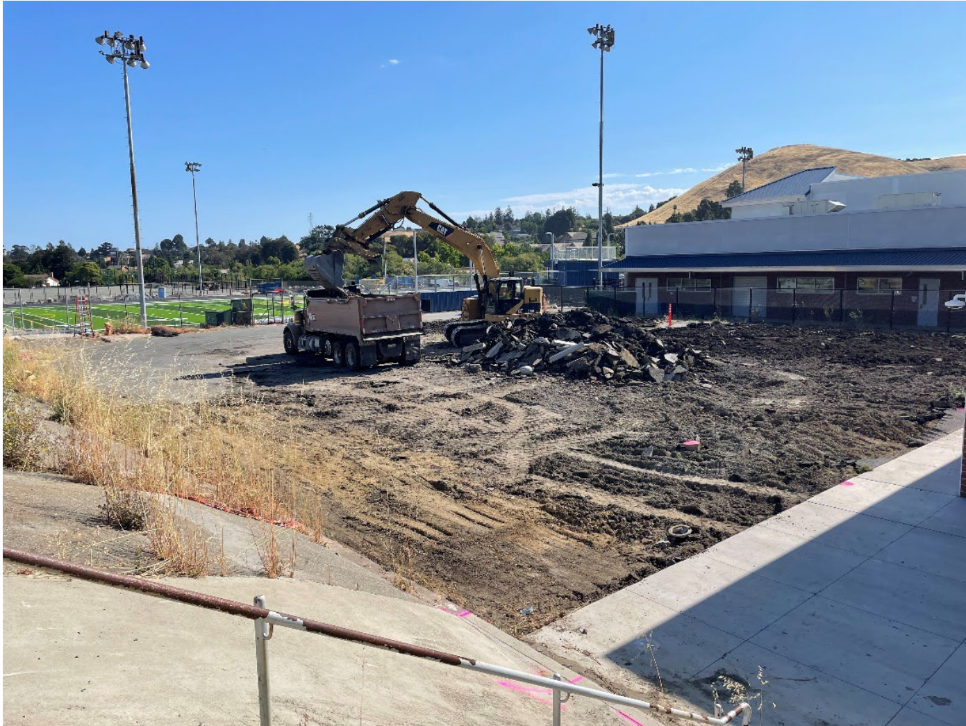
Removal of the portables
