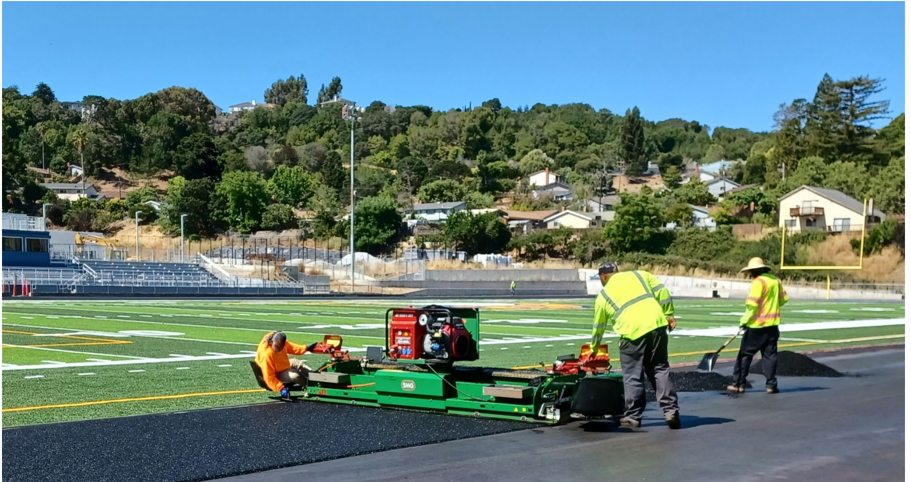
Track and Field Surface Replacement
