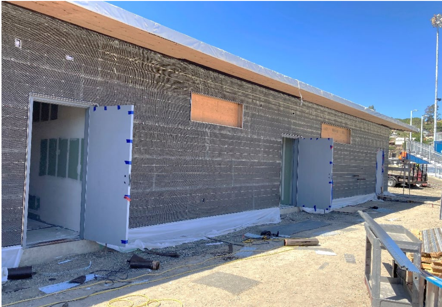
Field House competing metal lath preparing for stucco
