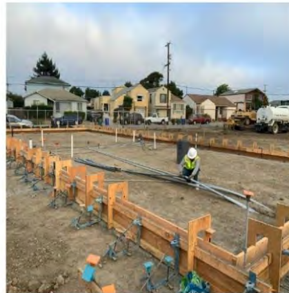
Running the utility lines
