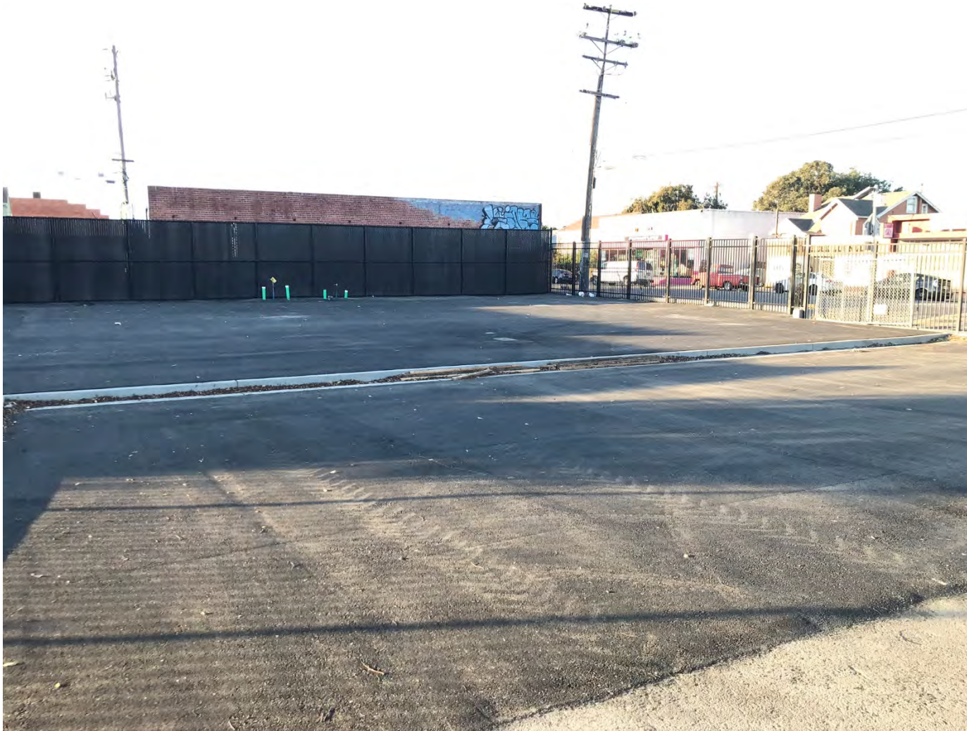
Paving and Fence for the New Health Clinic Location
