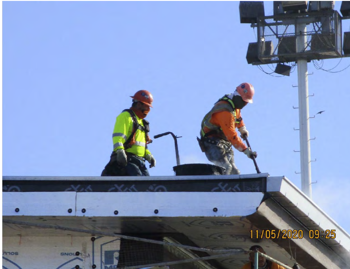
Roofing & Waterproofing Installation
