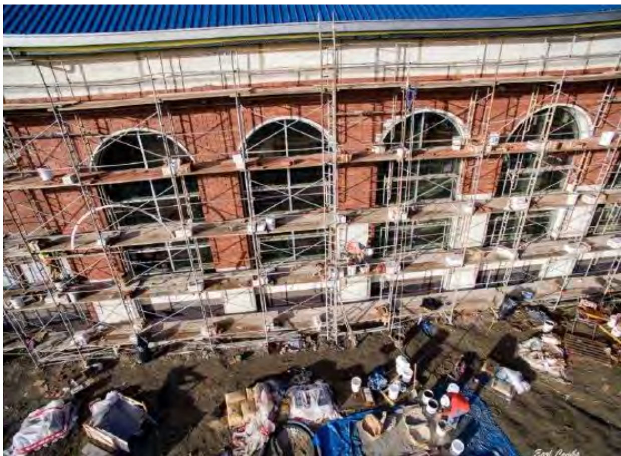
Pinole Valley High School - window installation
