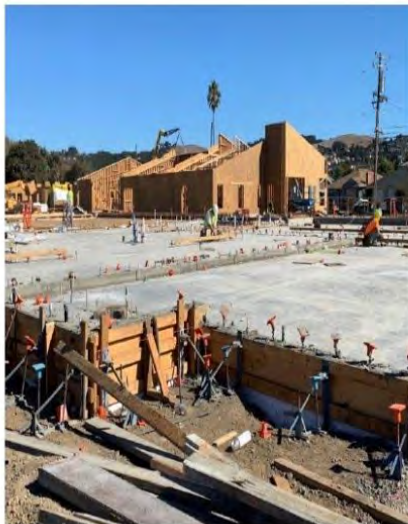
Cement slab work
