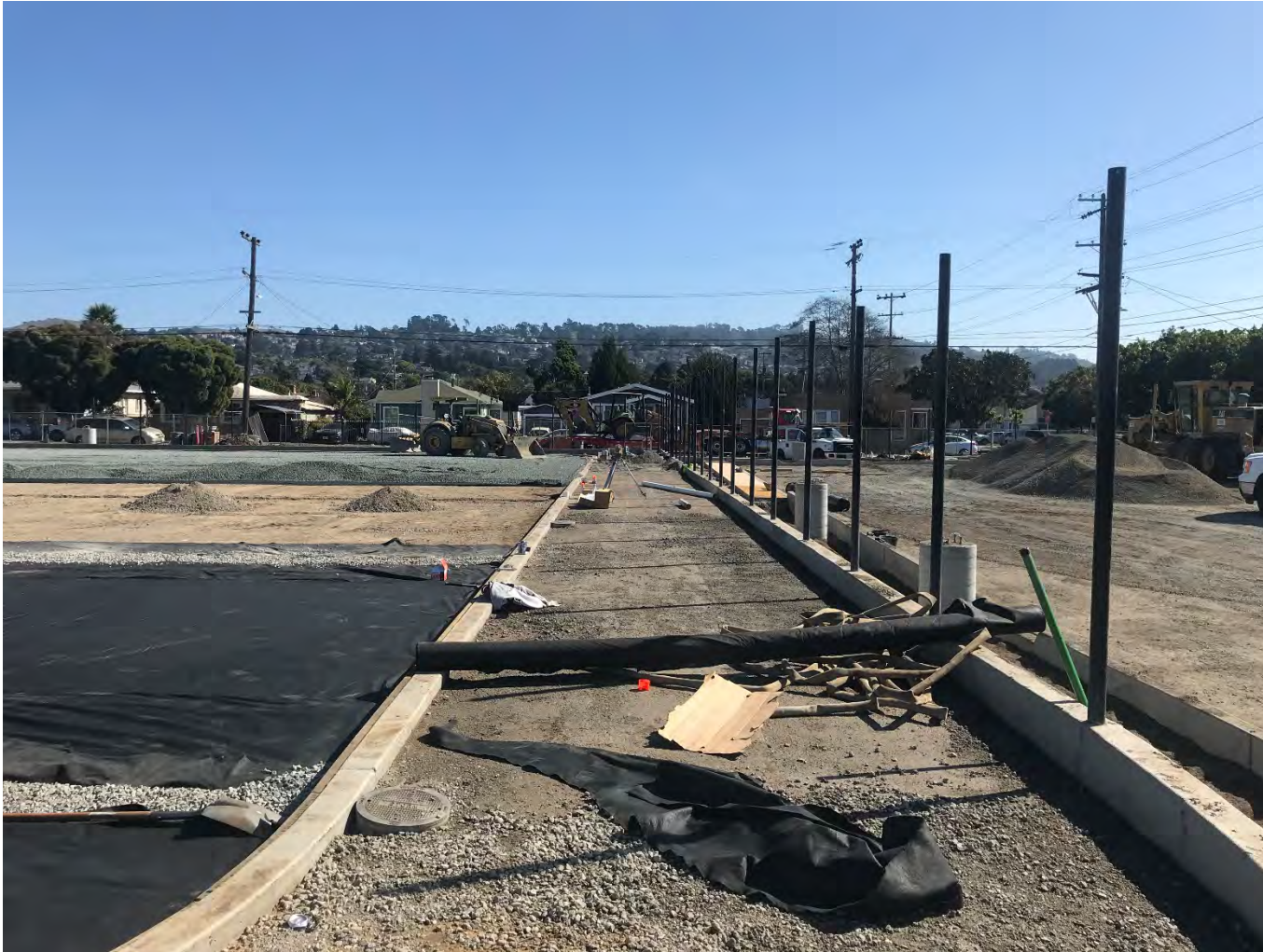
Turf Field & Track, South Parking
