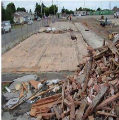
Demolition and clearing site
