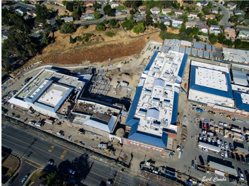
Pinole Valley High School - Construction 2018
