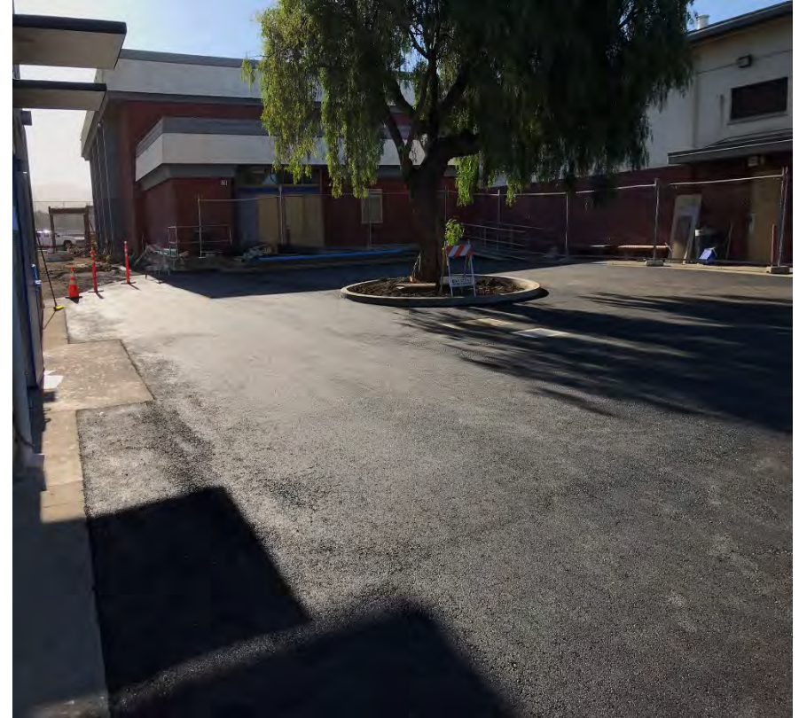
Science Quad AC Paving
