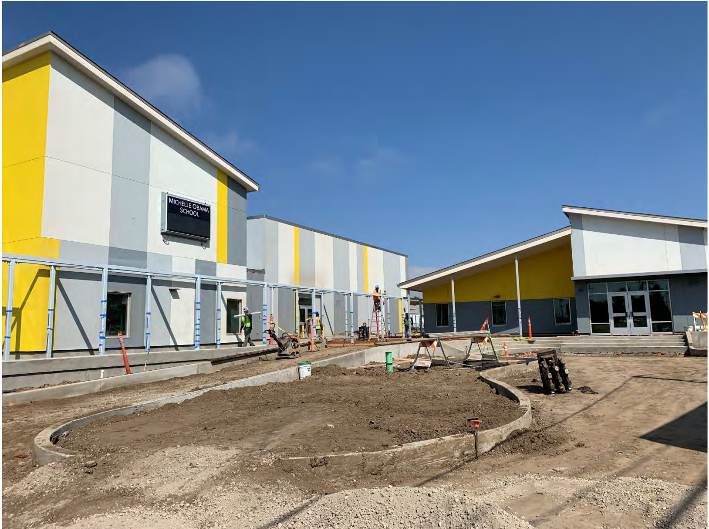
School Main Entry
