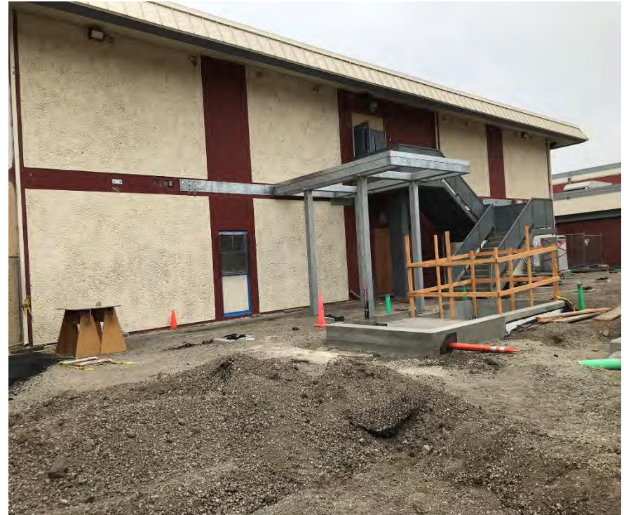
Elevator Landing Steel
