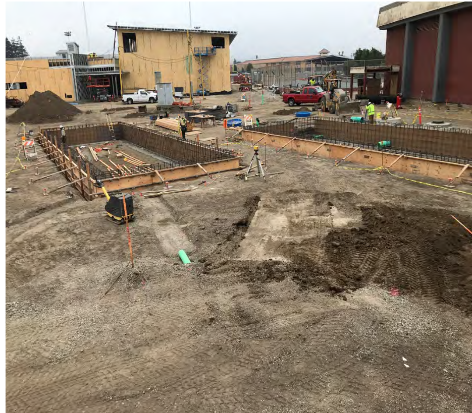
Bio Retention Walls
