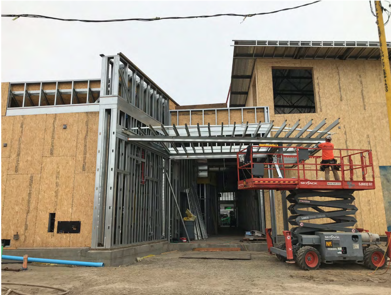
Gym Entry Canopy
