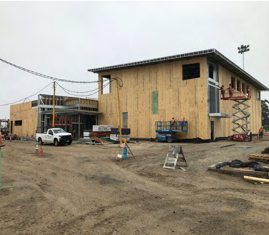
Gym Exterior Sheathing
