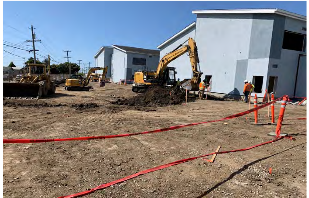
Excavate for Retaining Wall
