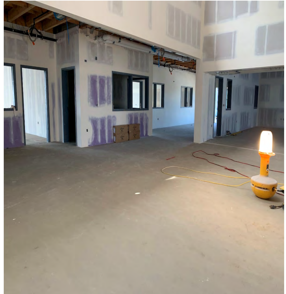
Learning Suites South Topping Slab
