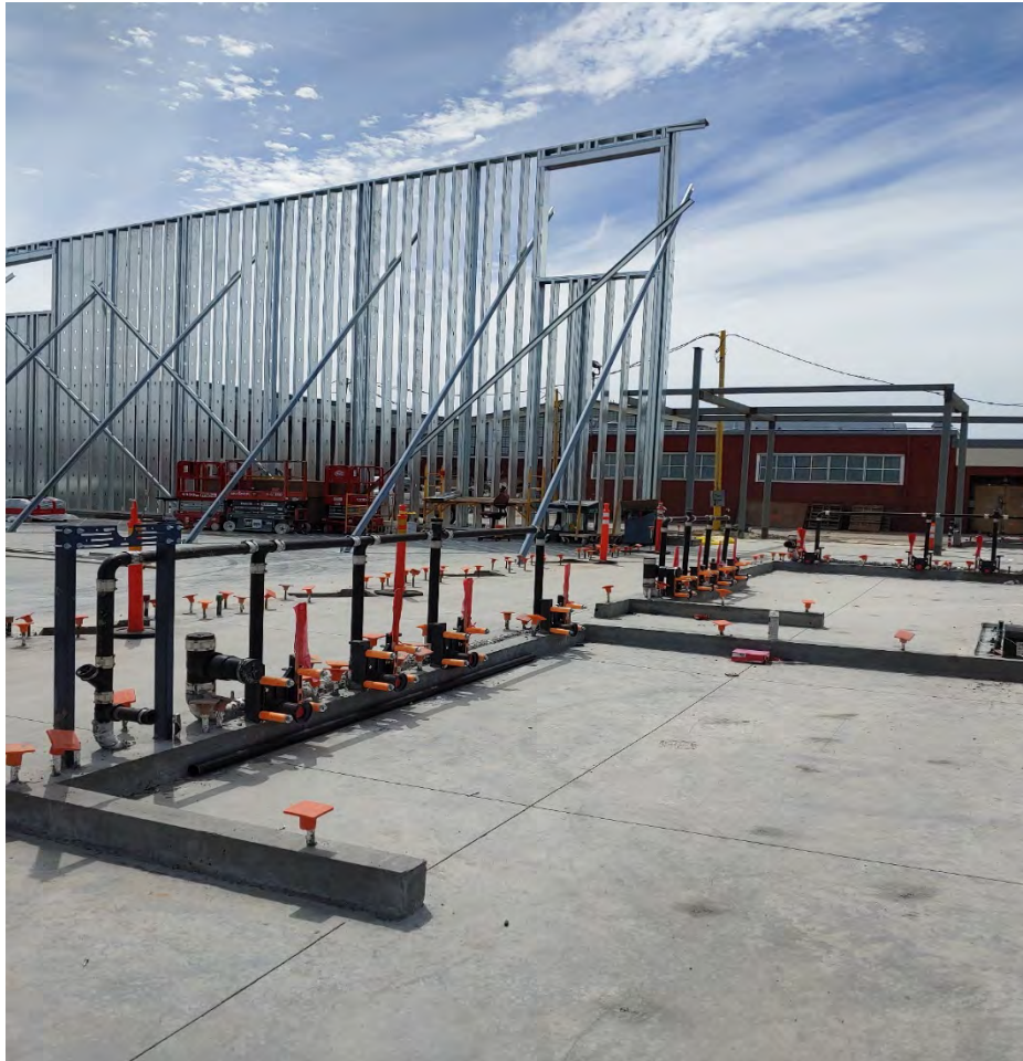
Gym Plumbing Rough-In
