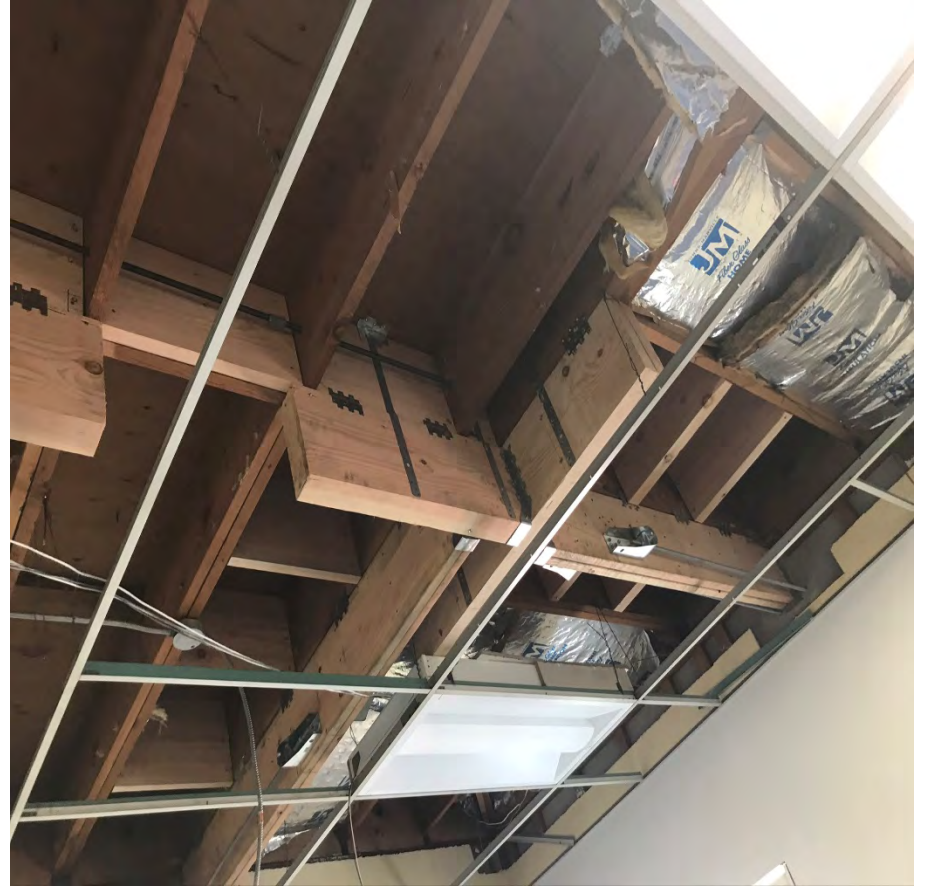
Seismic Blocking, Science Bldg.
