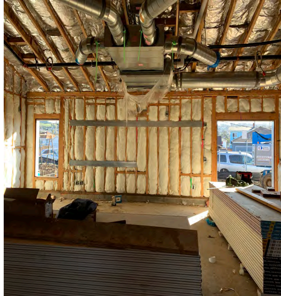
Library Insulation & Plaster
