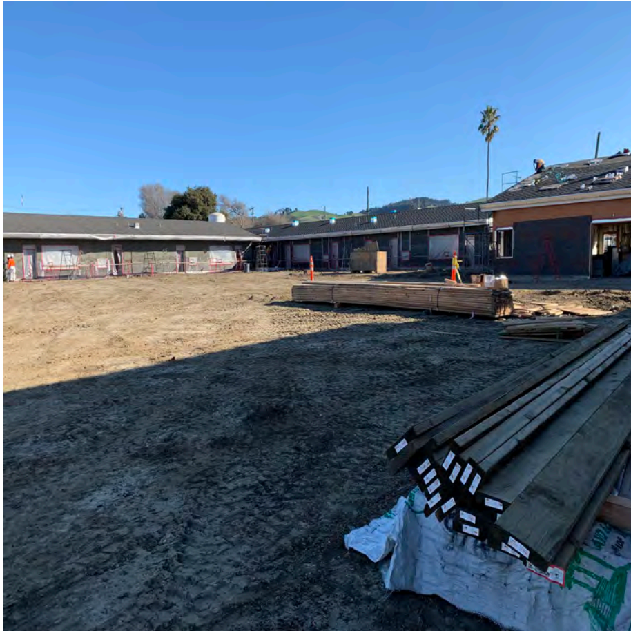
Admin Roof Shingle and Wall Lath
