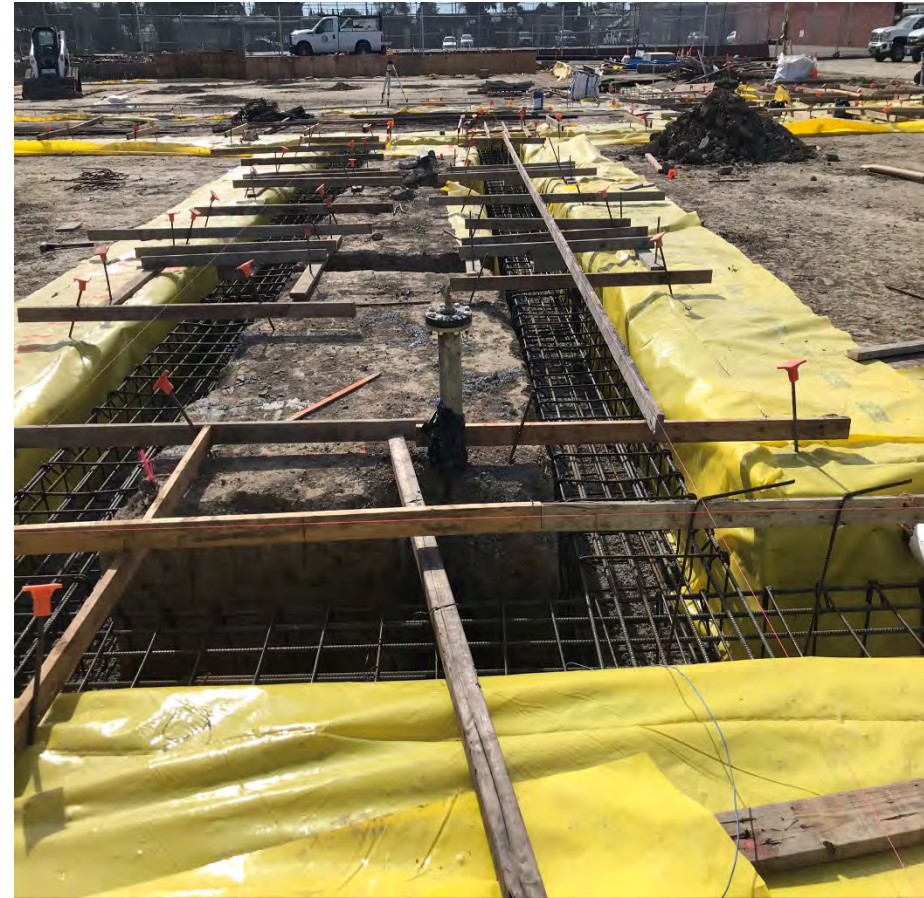
Gym Footing Rebar
