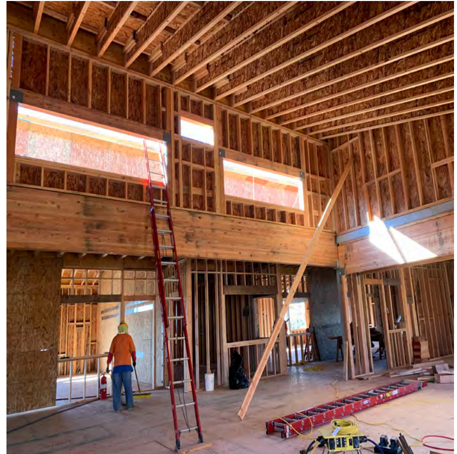
Learning Suite South 2 nd Floor Framing
