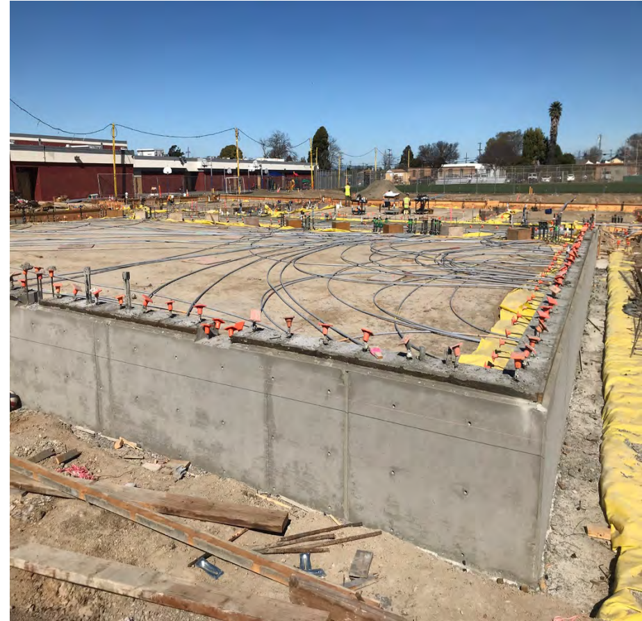
Gym Footing Stemwall
