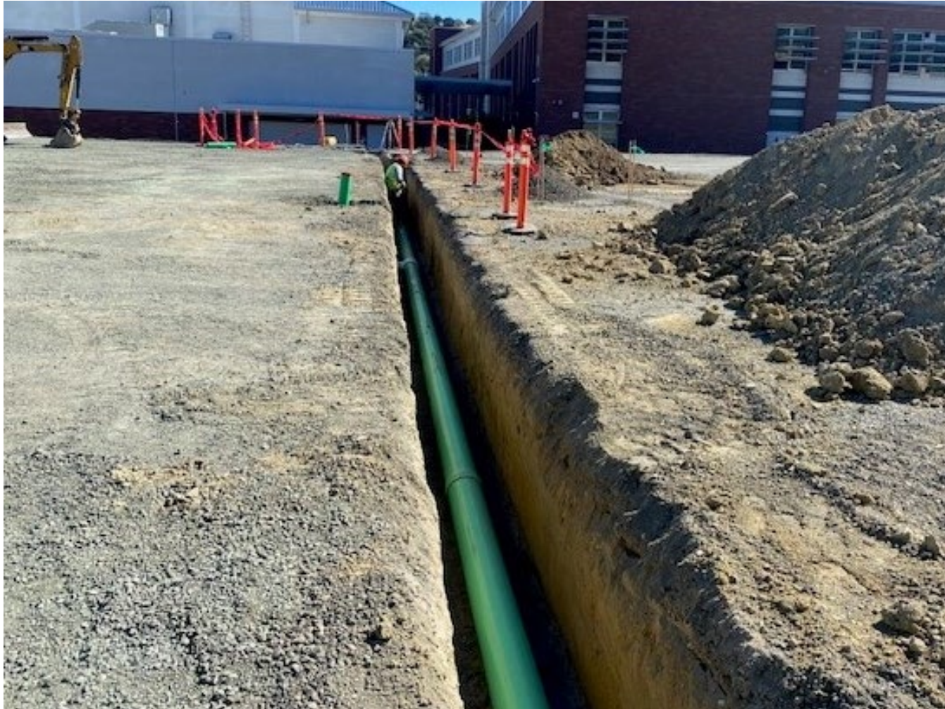
Subdrain installation
