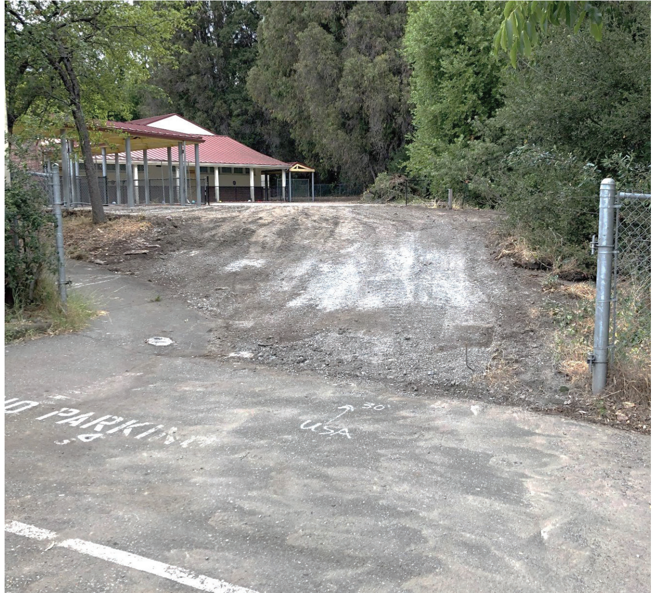
Late June – Cleared Path for Construction Equipment
