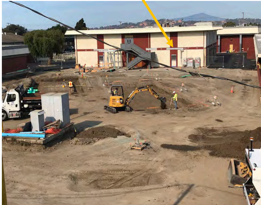
New Structural Support
