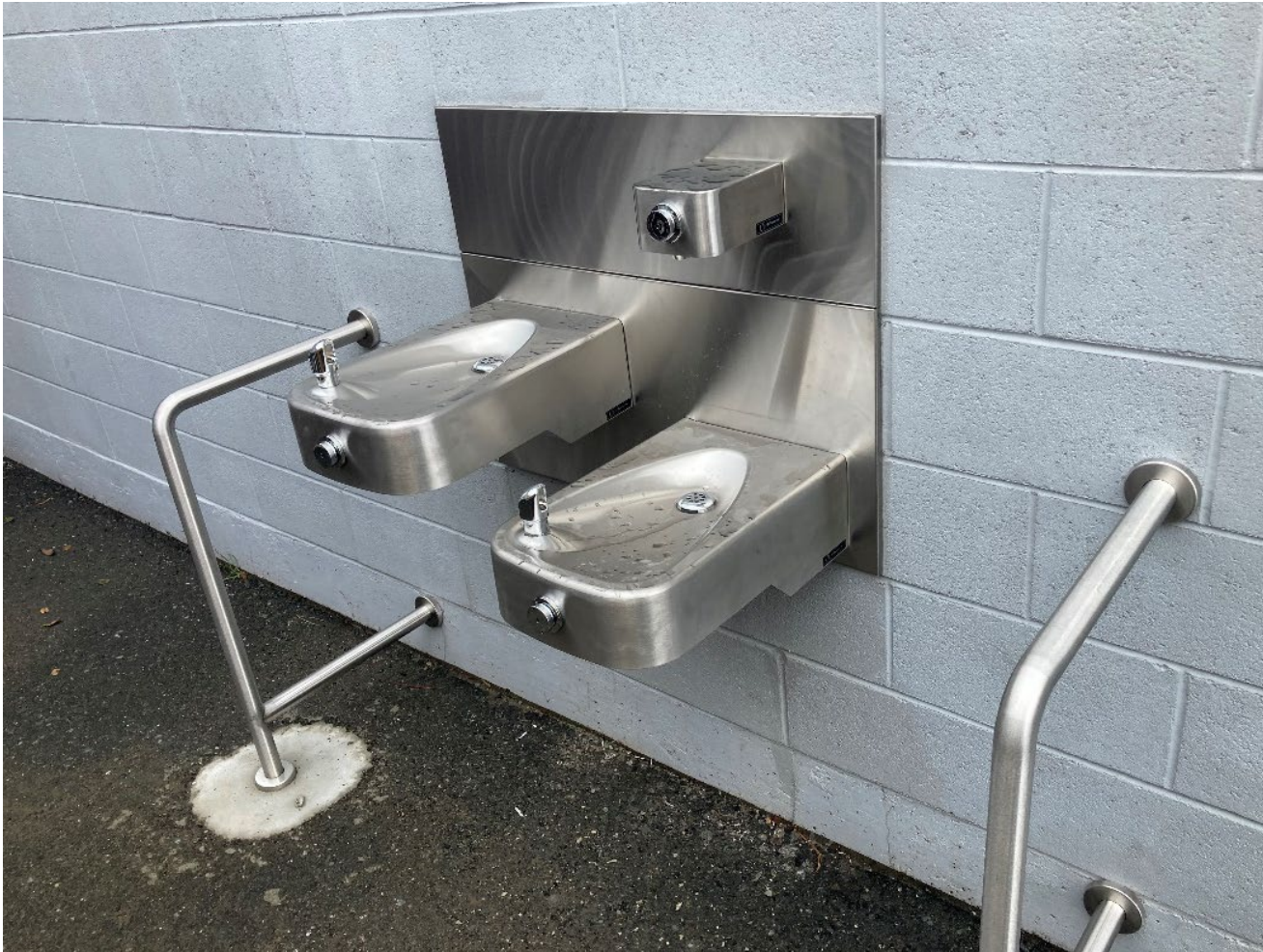
New Fixtures Installed at Existing Fieldhouse
