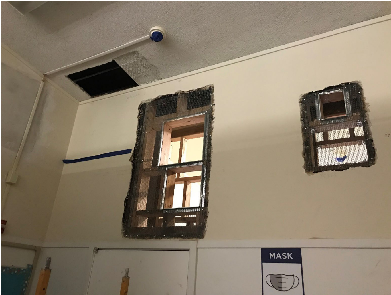
New wall penetrations for HVAC ductwork and plumbing feeds
