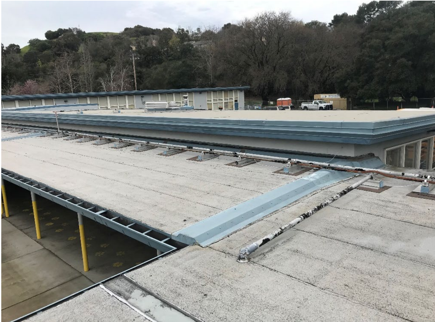
Roof and Existing Infrastructure Investigation
