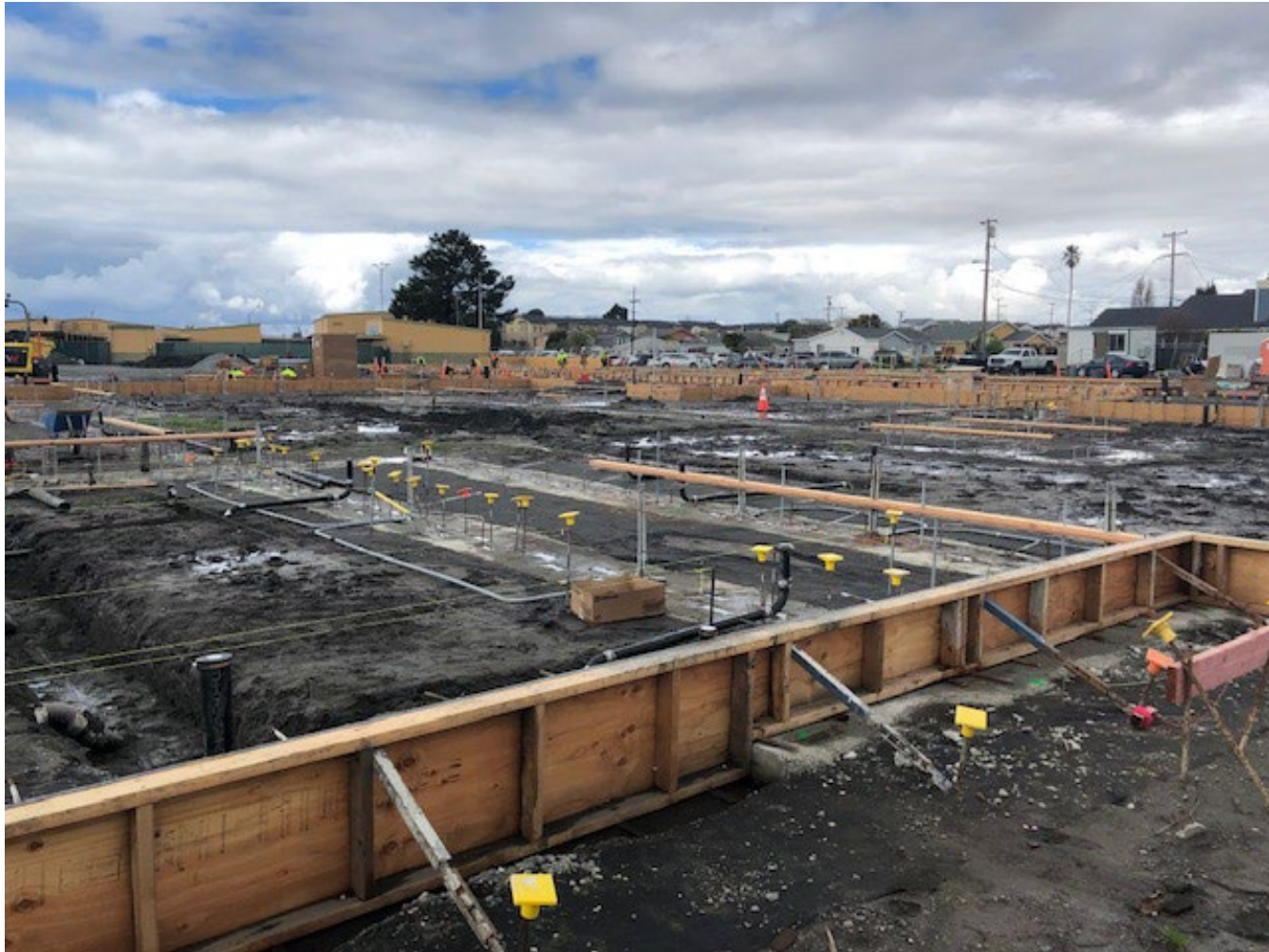
Slab Forming and Underslab Plumbing and Electrical at Building C
